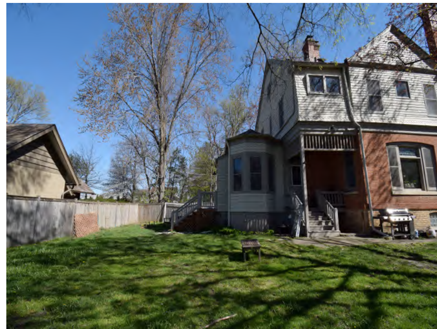
SIDE/ SOUTH FACADE
