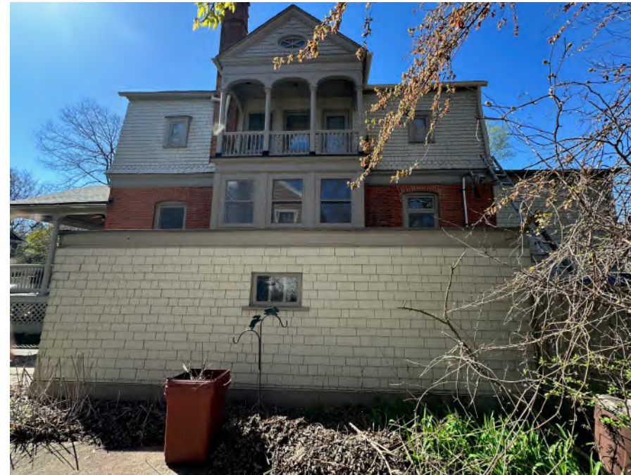
SIDE/ NORTH FACADE
