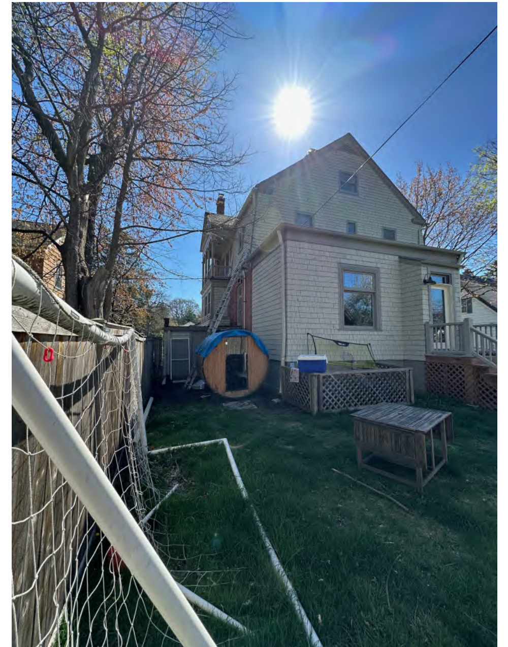
REAR/ WEST FACADE
