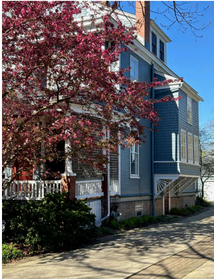
1618 ASHLAND-SIDE BAY BRACKETS
