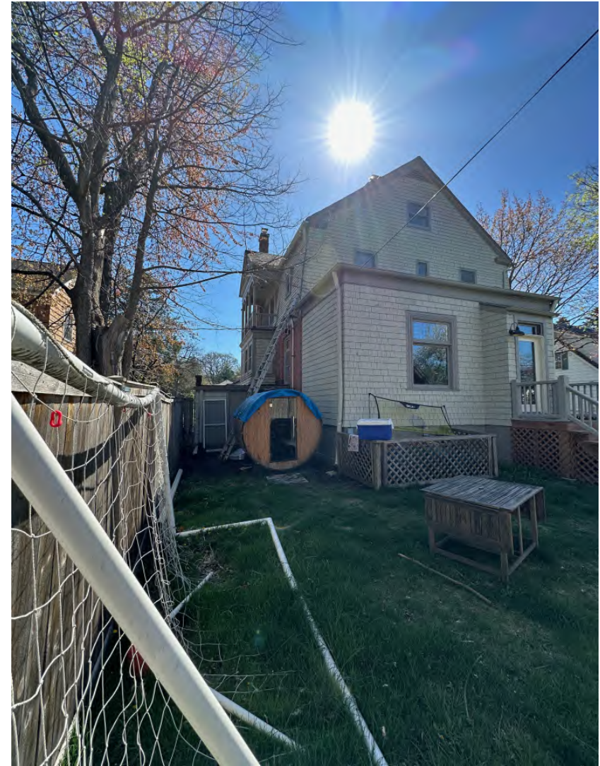
REAR/ WEST FACADE
