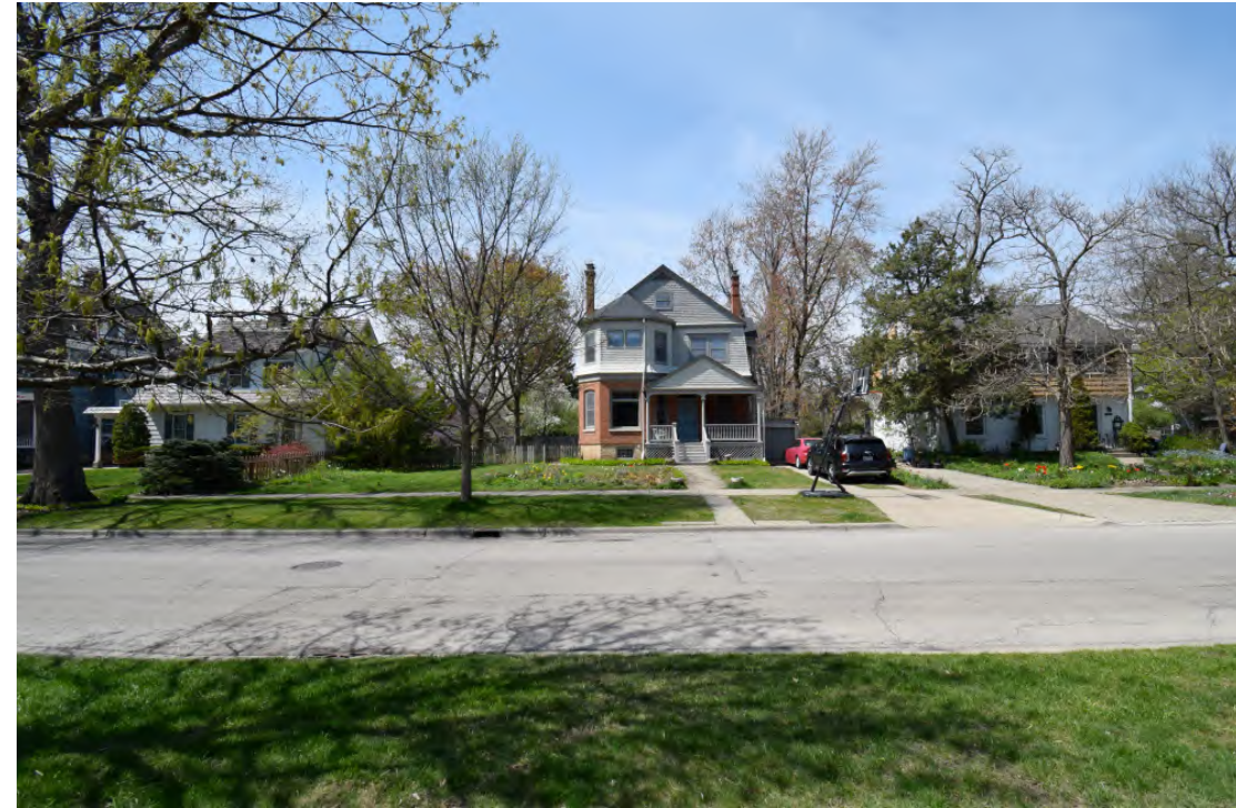
1618 ASHLAND-1624 ASHLAND-1630 ASHLAND-1632 ASHLAND
