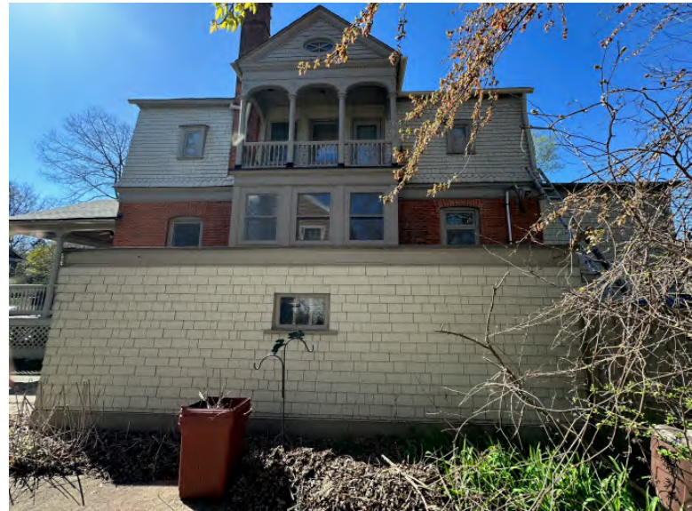
SIDE/ NORTH FACADE
