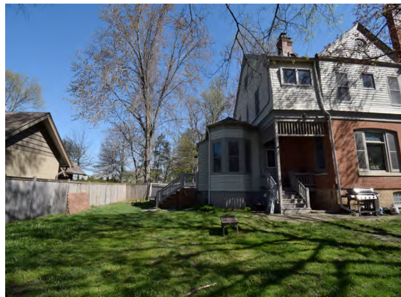
SIDE/ SOUTH FACADE
