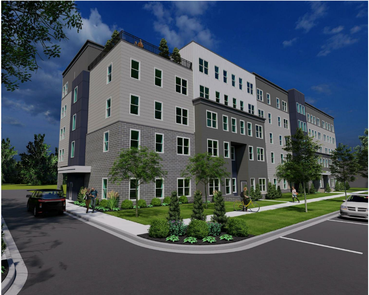
South Boulevard Shores 504 - 514 South Blvd. Evanston, Illinois
