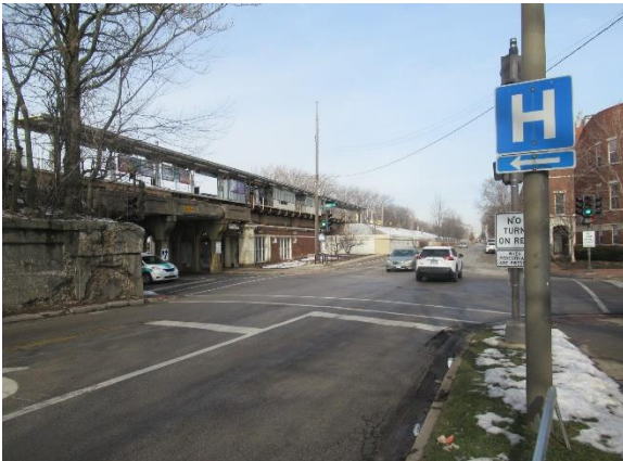
North on Chicago Avenue (Photo Taken on February 6, 2023)
