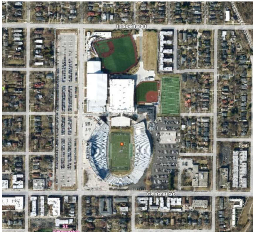
1501 Central Street - aerial
