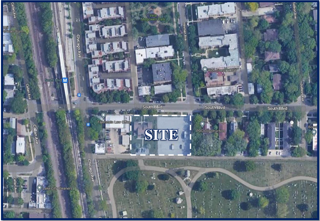
Aerial View of Site
