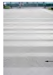
2 CAST-IN-PLACE CONCRETE-ACID ETCH
