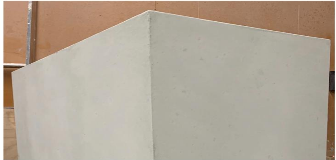
Sack Finish Concrete
