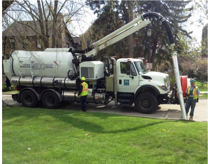
Sewer Division staff operate a sewer cleaning truck to remove debris from a catch basin.
