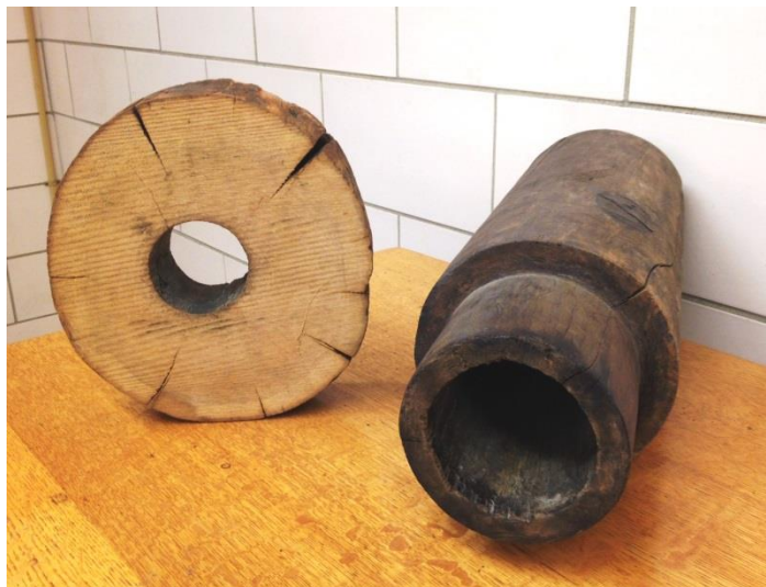
Pieces of wood water main from Evanston's original water distribution system.
