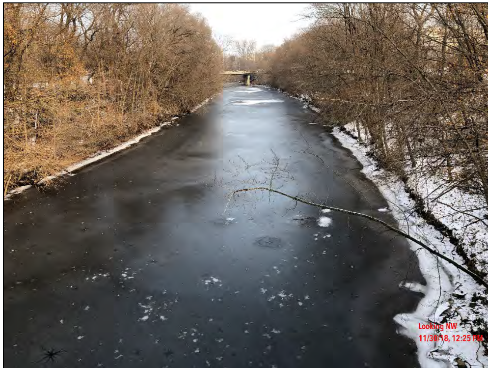
Photo 28: Looking upstream, channel in good condition.
