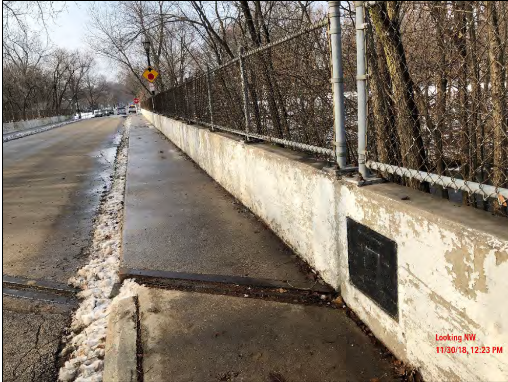
Photo 7: Typical sidewalk, parapet and chain link fence configuration.
