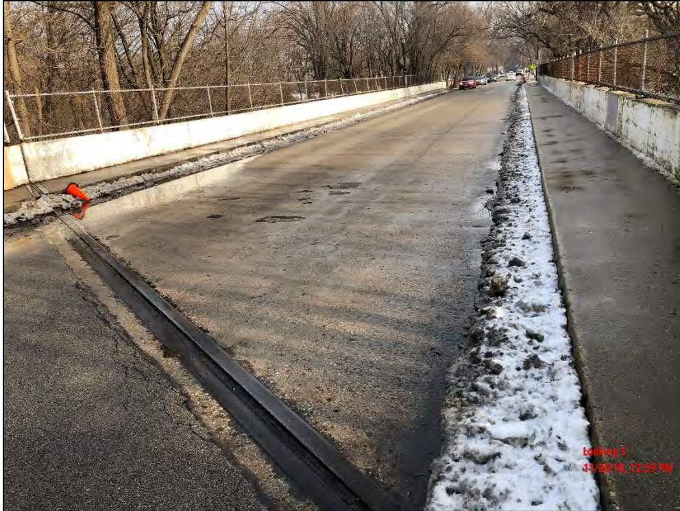
Photo 3: Overall top of bridge deck.
