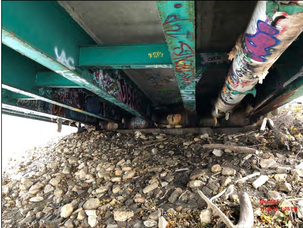
Photo 19: Overall East abutment Elevation. Similar Configuration for West abutment.
