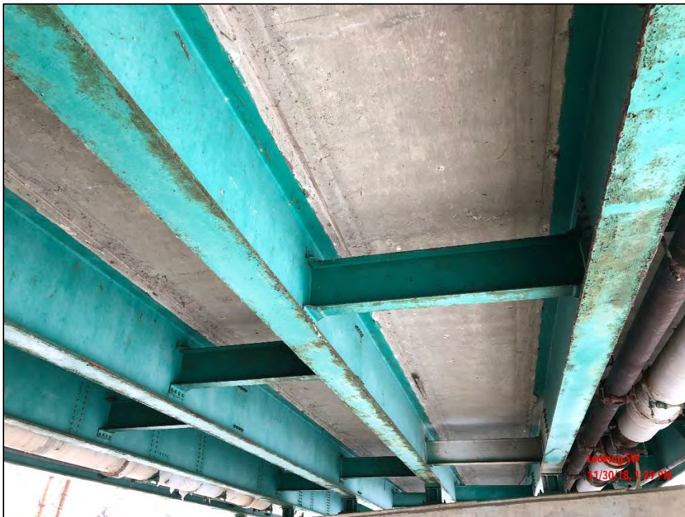
Photo 16: Deck underside East Span; similar condition to West Span.
