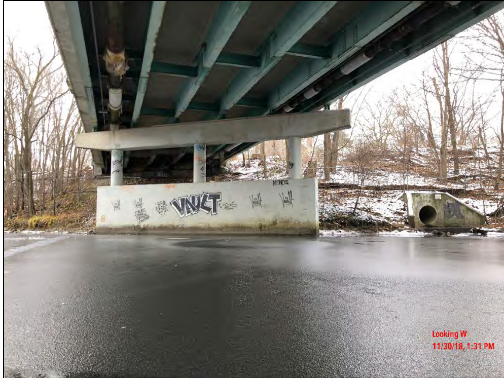
Photo 21: West pier elevation.
