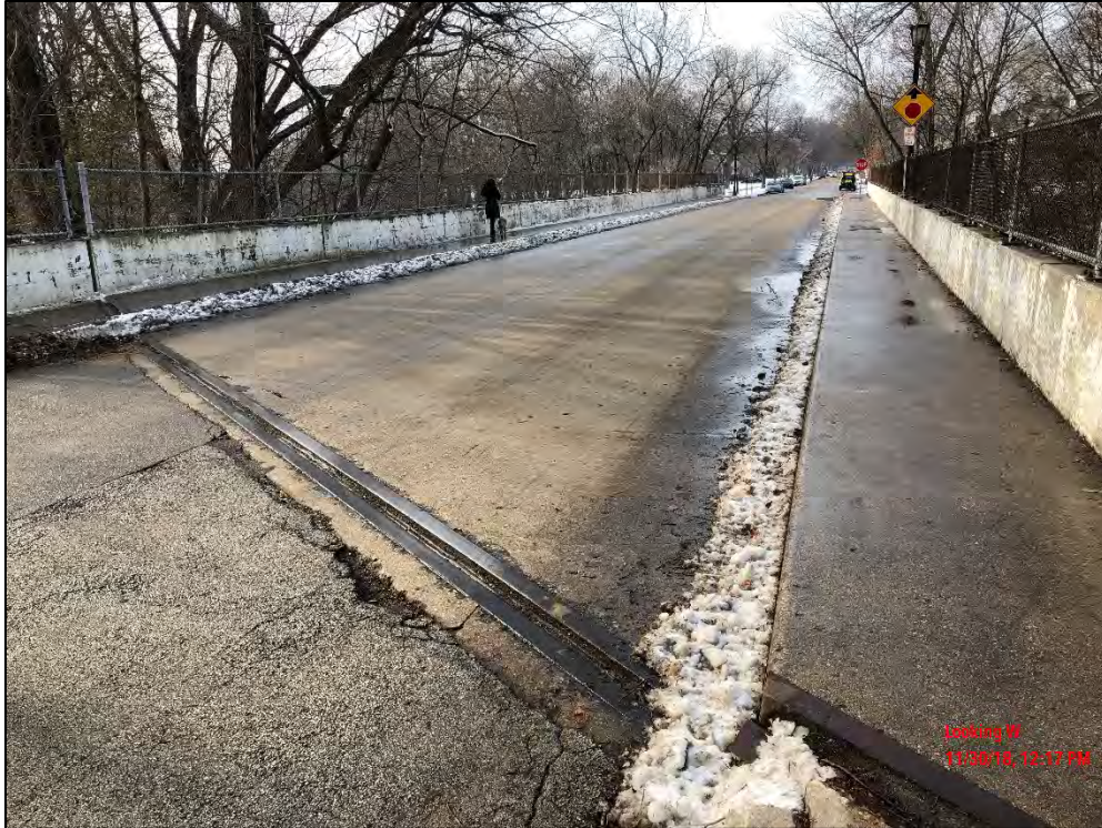
Photo 1: Overall top of bridge.
