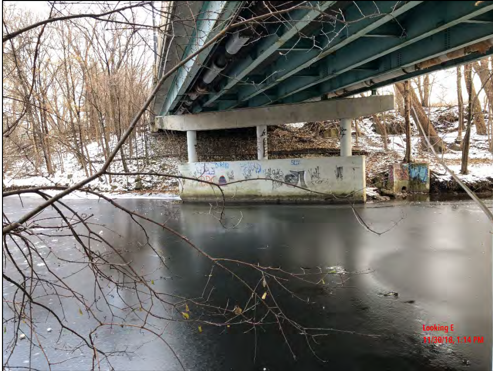
Photo 25: East Pier Elevation.
