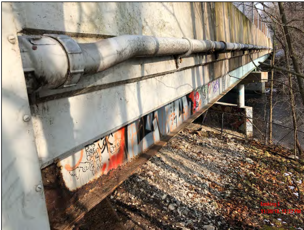
Photo 30: South Parapet noted with electrical conduit. Connection is in good condition.
