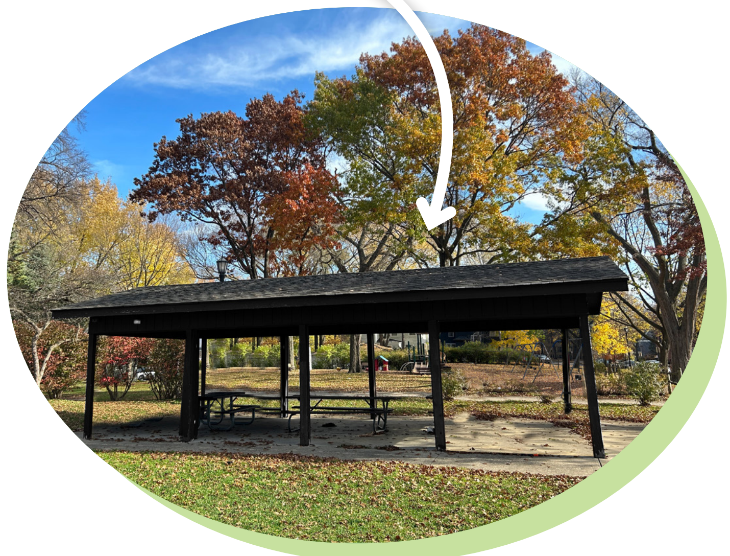
Option: Dark Painted Wood with Panels Removed to create Open Air Structure
