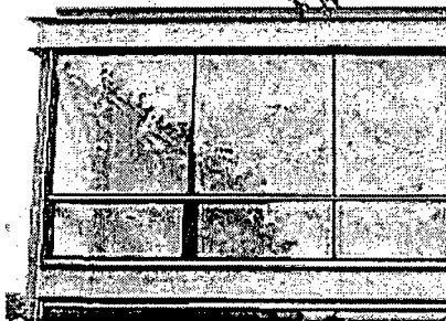
WINDOW WALL: High performance double insulated glass units with clear anodized aluminum or grey color fiberglass composite frame
