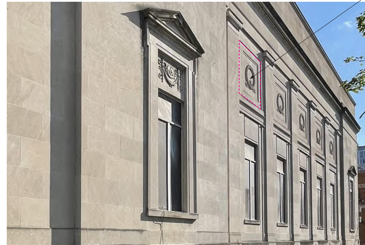
EXISTING CONDITION: SOUTH FACADE
