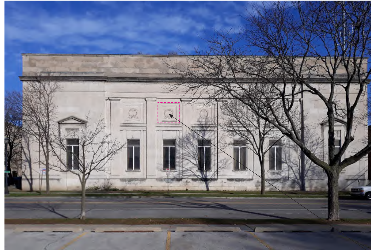
EXISTING CONDITION: SOUTH FACADE
