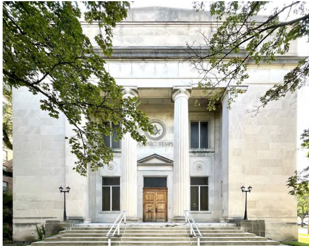
EXISTING CONDITION: WEST FACADE
