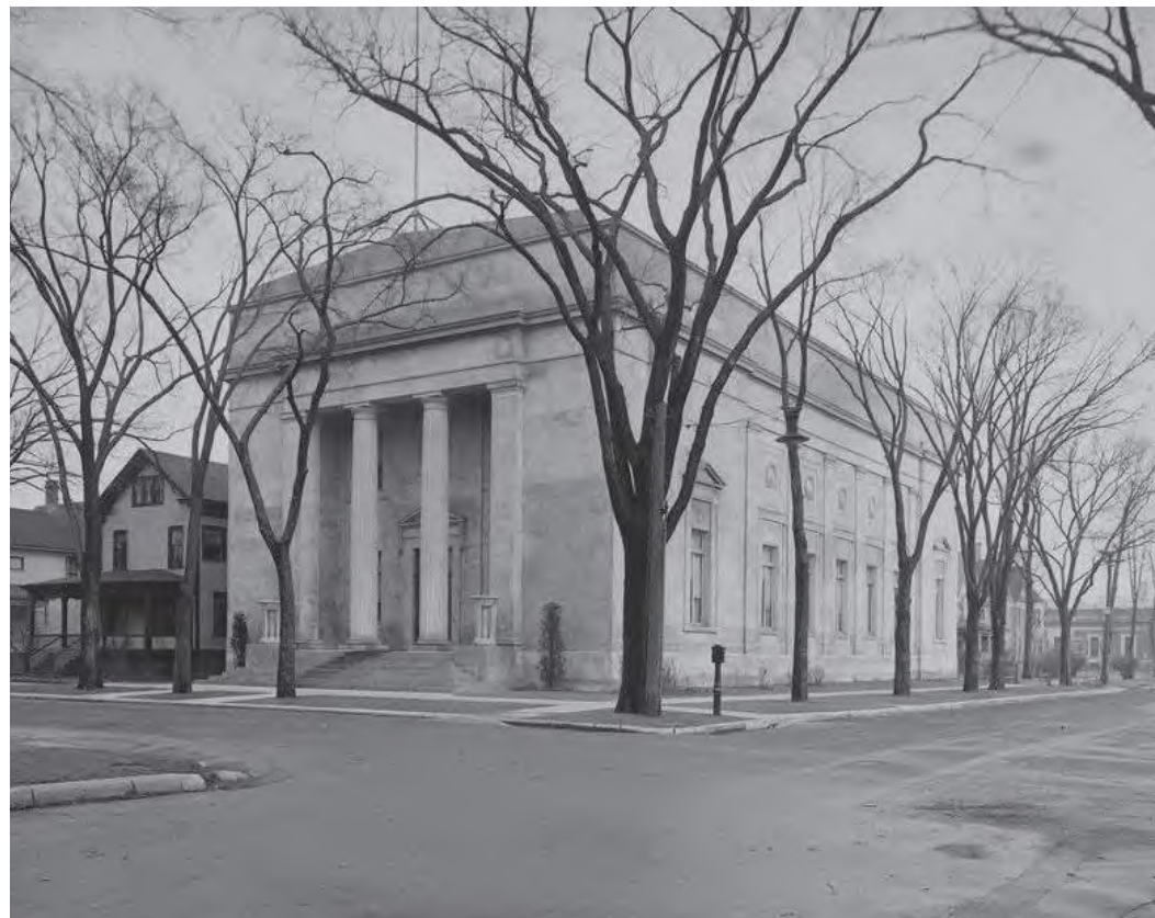
HISTORIC IMAGE : VIEW FROM SOUTHWEST
