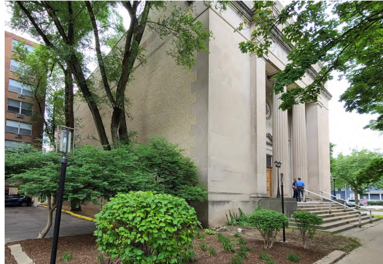
EXISTING CONDITION: VIEW FROM NORTHWEST
