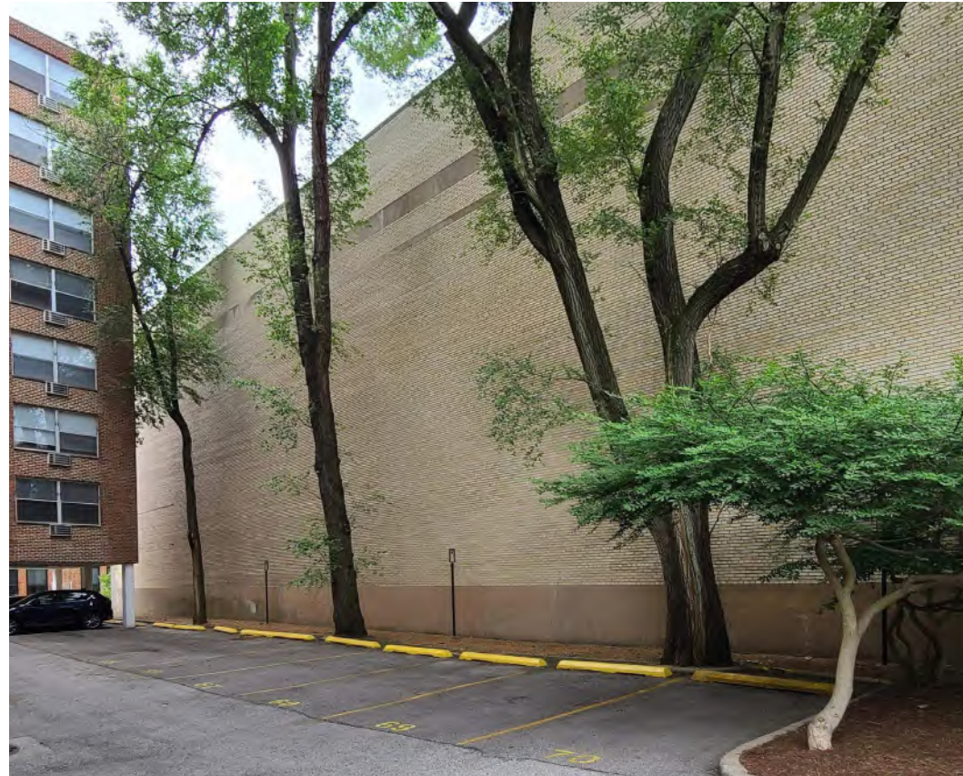
EXISTING CONDITION: NORTH FACADE
