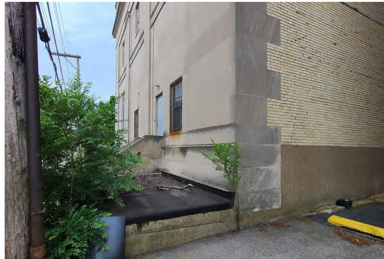
EXISTING CONDITION: VIEW FROM NORTHEAST
