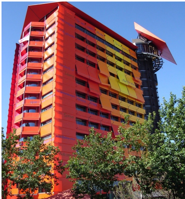
Strategy 1: Use external solar or security screens, shades or grilles, like these motorized solar shades.
