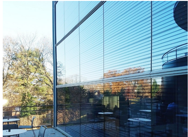
Strategy 2: Use bird-friendly glass. Here, dark, reflective glass incorporates a pattern of fritted lines visible to birds.
