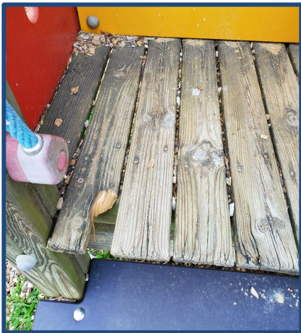
Fitzsimmons Park - Failing Wood Playstructures
