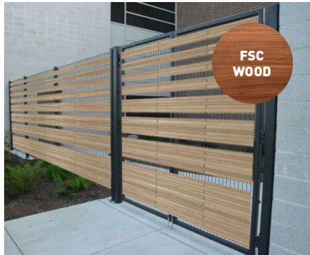
ADD ALTERNATE: WOOD PANELS FSC-CERTIFIED CUMARU WOOD, 2" X 6" PLANK, CUSTOM FABRICATED BY GC PATTERN A: HORIZONTAL, SOLID BOTTOM, GRADIENT TOP
