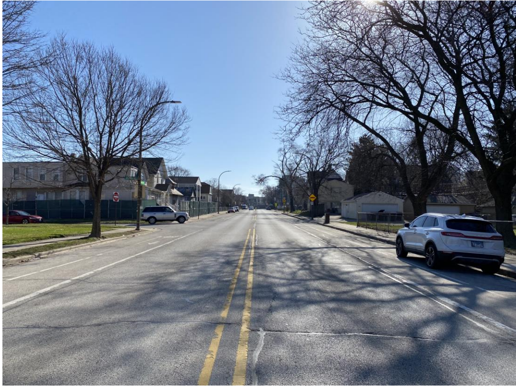
STREET VIEW EMERSON STREET, LOOKING EAST
