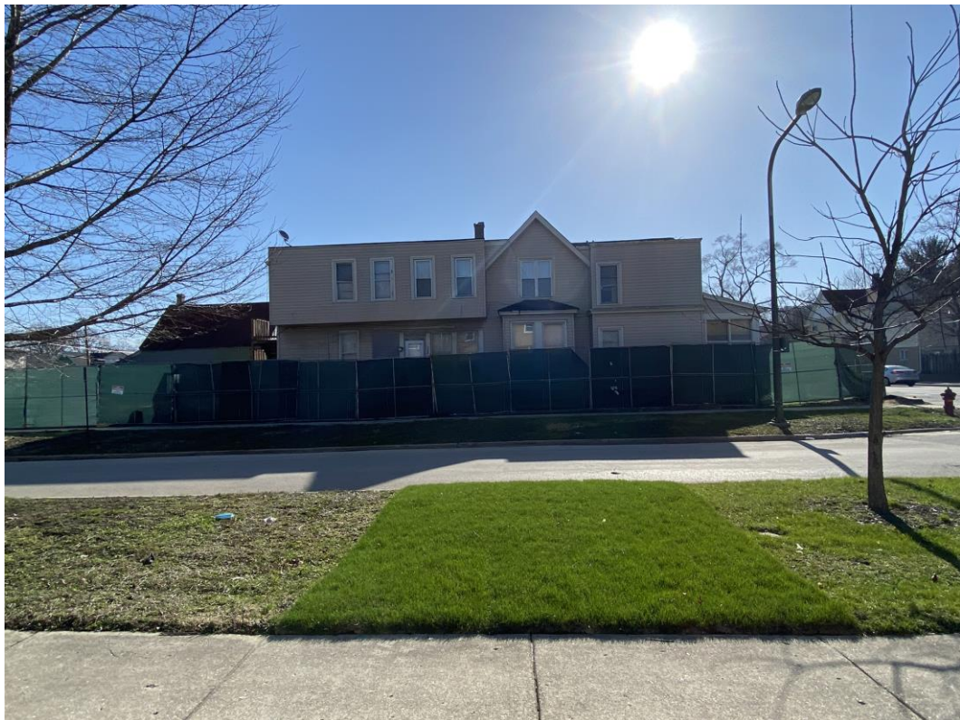
LOOKING EAST FROM WEST SIDE OF JACKSON AVENUE
