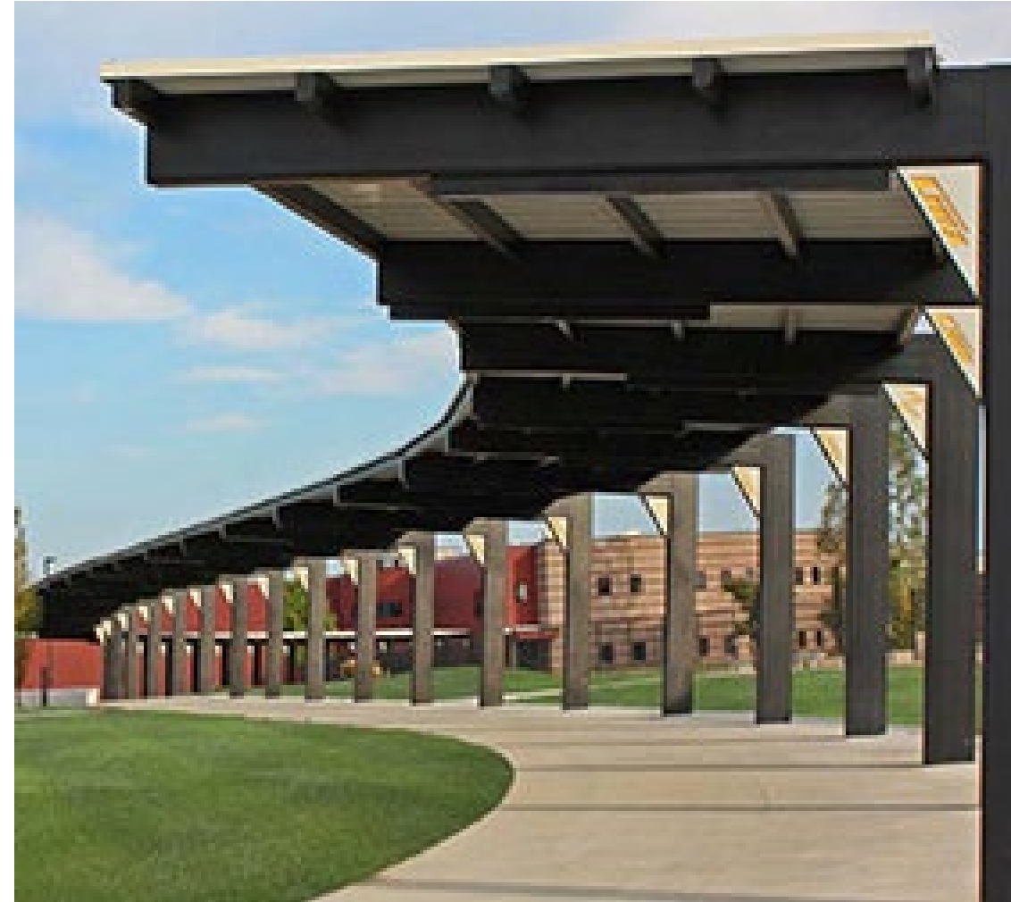
POLIGON – SHADE STRUCTURE
