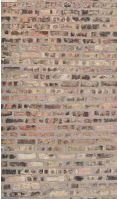
EXISTING COMMON BRICK
