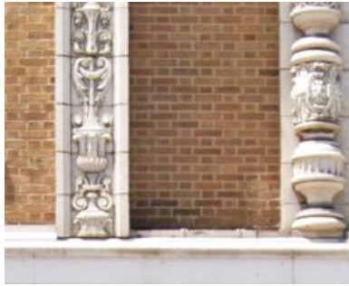
EXISTING FACE BRICK AND TERRACOTTA
