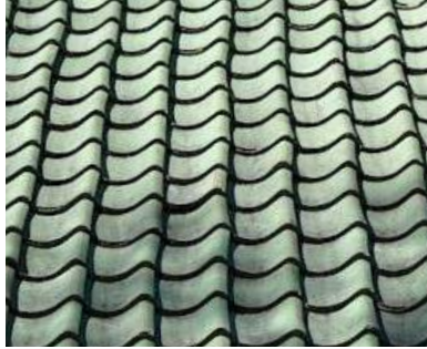
EXISTING TILE ROOF
