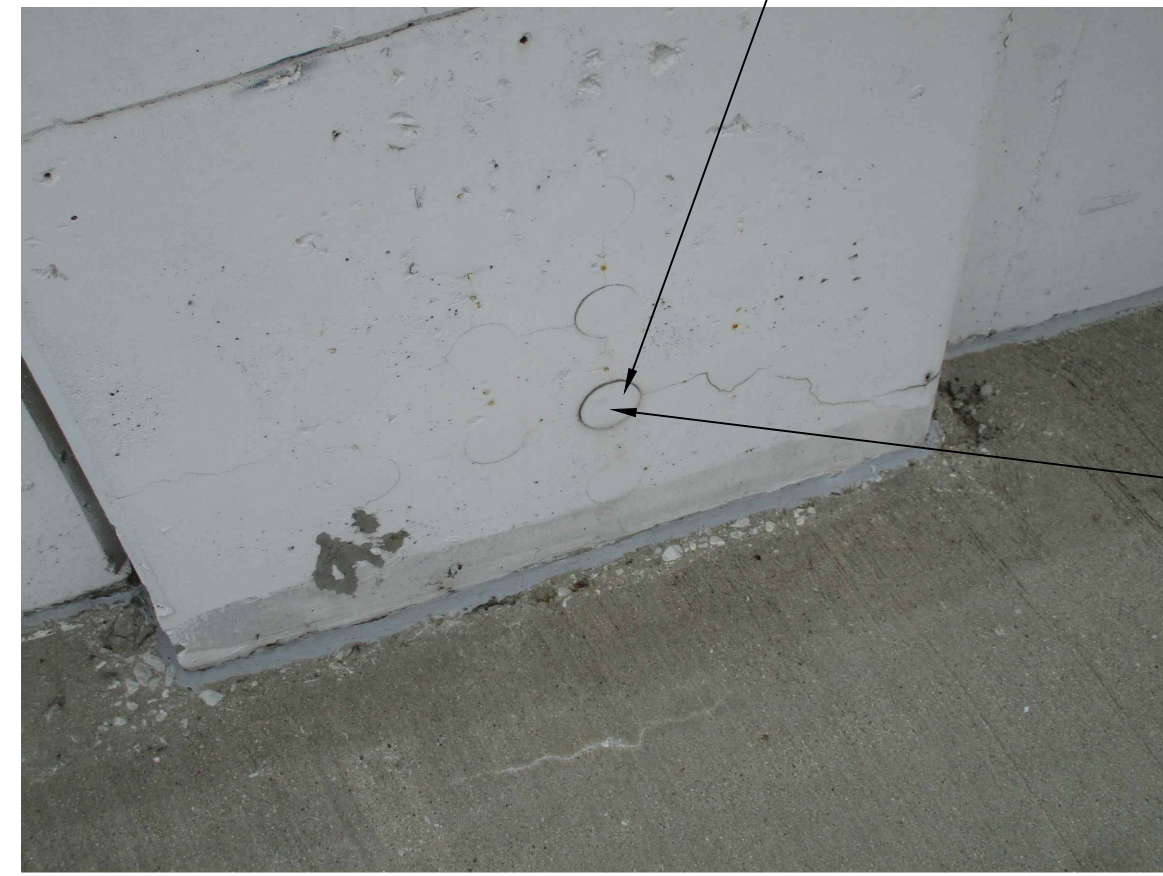
2 POST-TENSIONED GROUT POCKET REPAIR NOT TO SCALE
