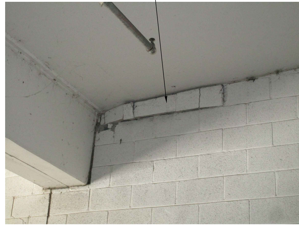
1 CMU REPAIRS AT DAVIS STREET EXIT RAMP NOT TO SCALE
