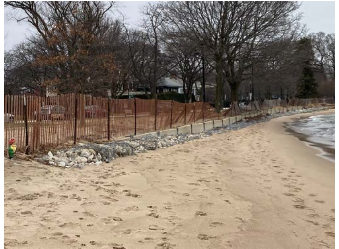
Image 2: Exposed h-pile and concrete wall
