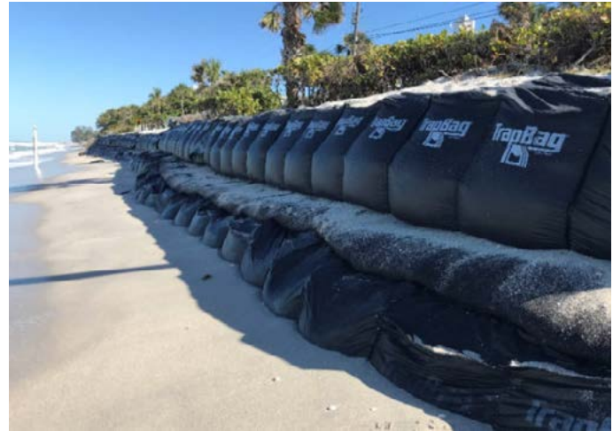
Image 7-1: Trapbag - Sand-filled & Planted
