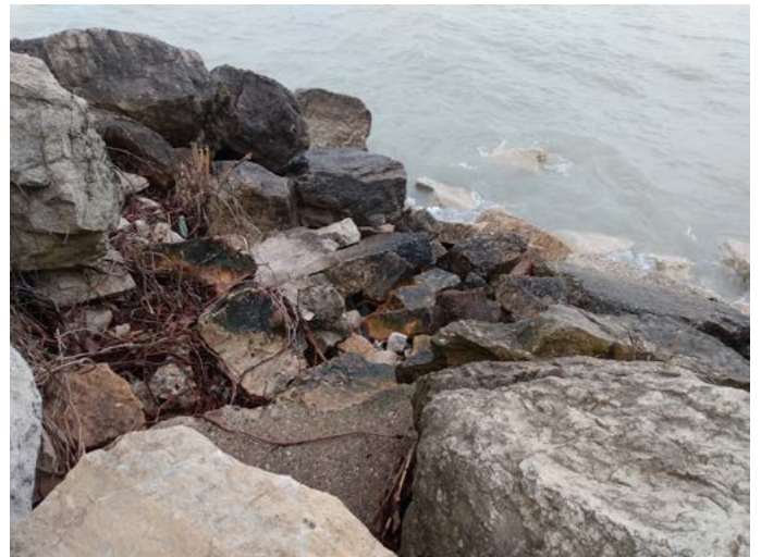
Image 4: Varying stone sizes along revetment slope
