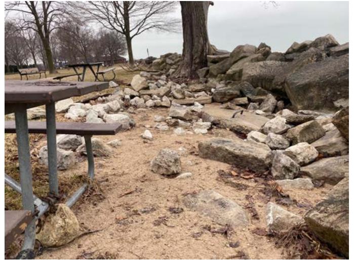
Image 2: Significant landscape damage and displaced stone
