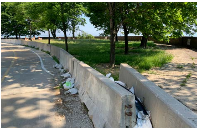
Image 7-2 Temporary Concrete barriers at 67th Street, Chicago
