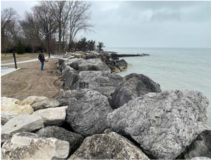
Image 1: Varying width in crest protection
