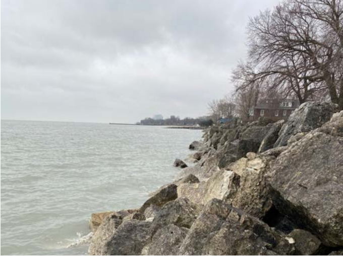
Image 1: Revetment stone stacked at near vertical slope
