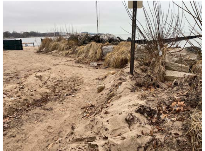
Image 2: Sand transport into driveway
