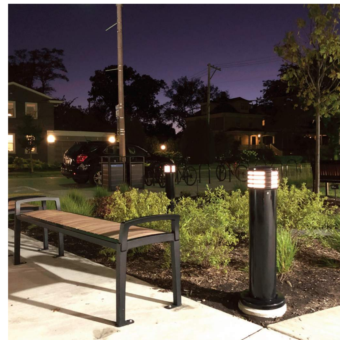
G-6: LED Lighting
