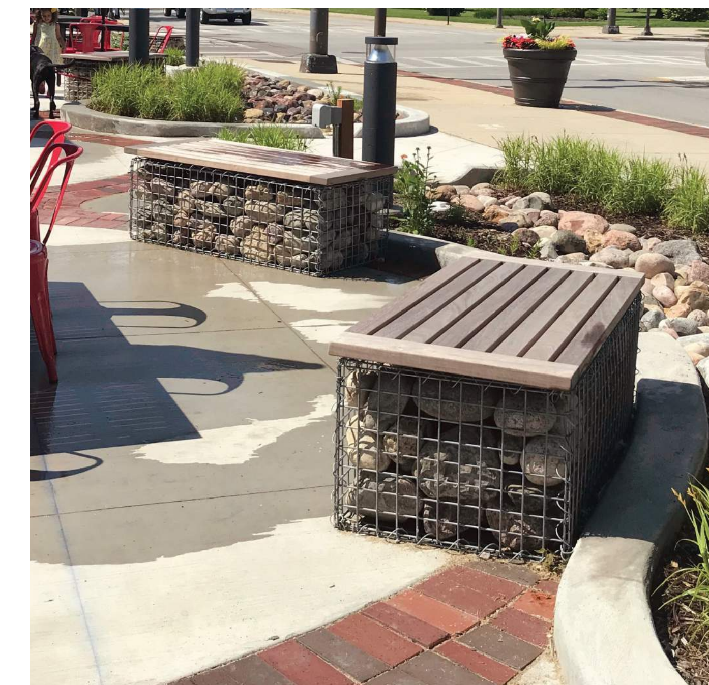
G-8: Gabion Benches
