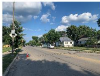
Road tubes on Simpson St. near the control site at Twiggs Park (Monitoring Station 5).
