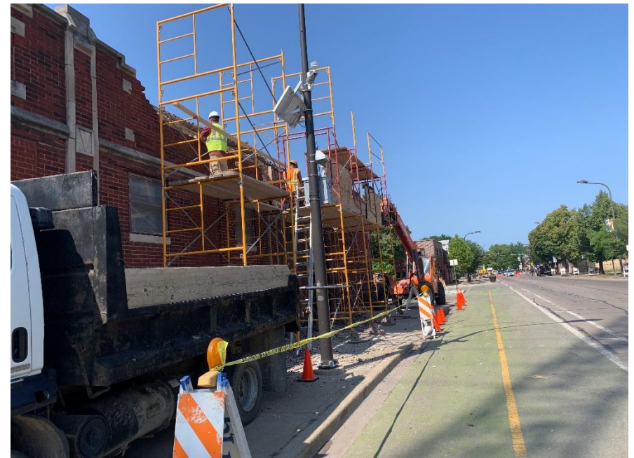
Reason #10 – Tuckpointing brick facade nearby Site 4 on Church St.
