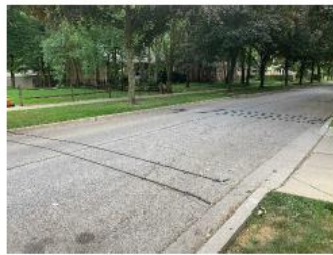
Road tubes on Ashland Ave. near Monitoring Station 2.
