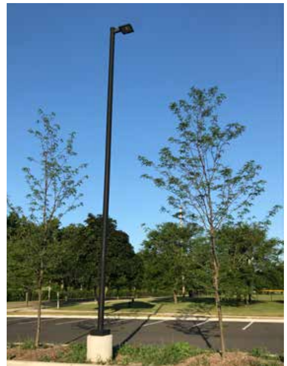
Figure 3.6: Parking Lot Lighting Unit
