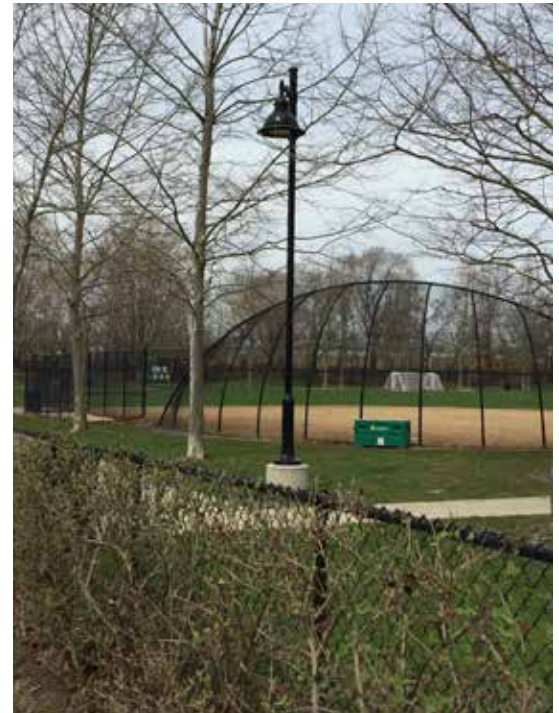
Figure 3.5: City of Evanston Bike/Pedestrian Pathway Lighting Unit
