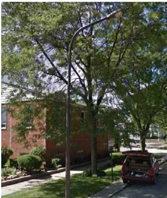
COBRA HEAD METAL HALIDE (ROADWAY)
