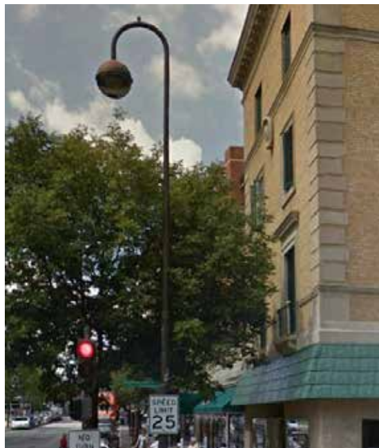
GLOBE TYPE HIGH PRESSURE SODIUM (ROADWAY)
