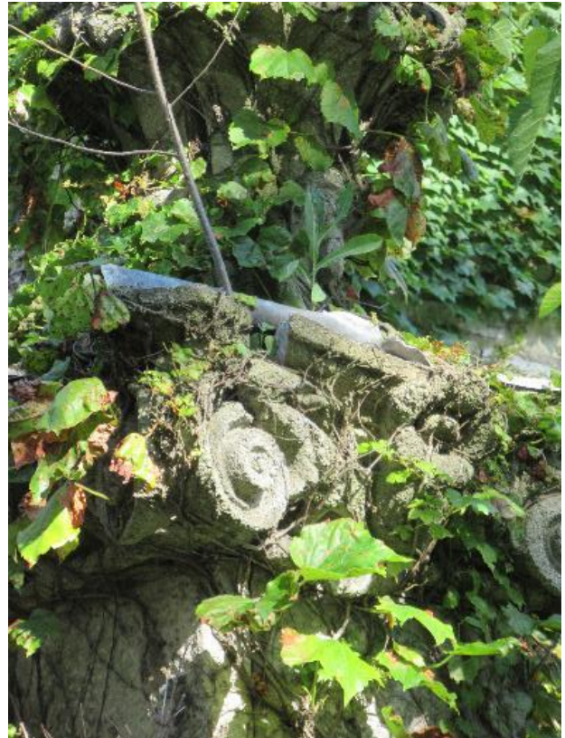
Figure 35. Flashing between urn and ornamental cast stone capital east facade
