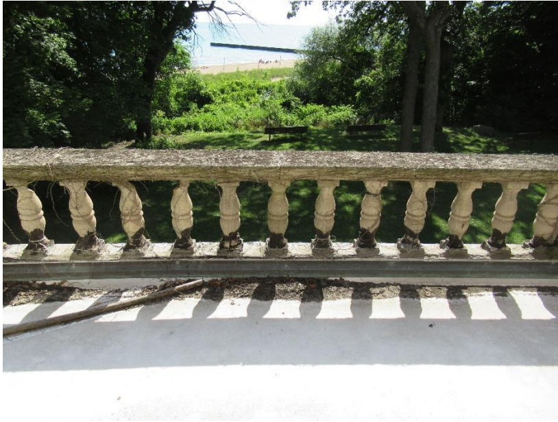
Figure 25. Limestone balusters at second floor balcony above sun room
