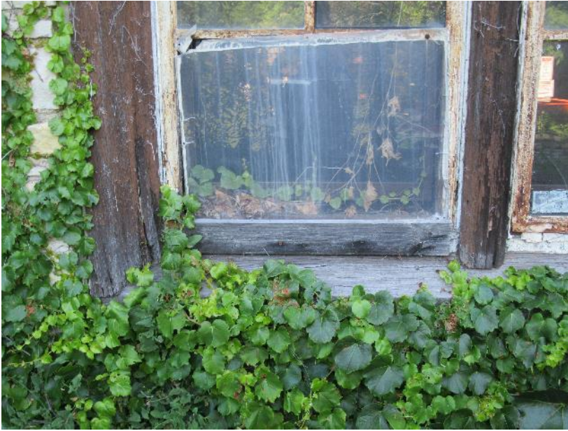
Figure 29. Window wood jambs and glazing at west facade
