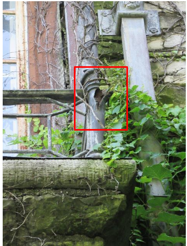
Figure 34. View of Juliette balcony (left) and cracked cast iron (right)
