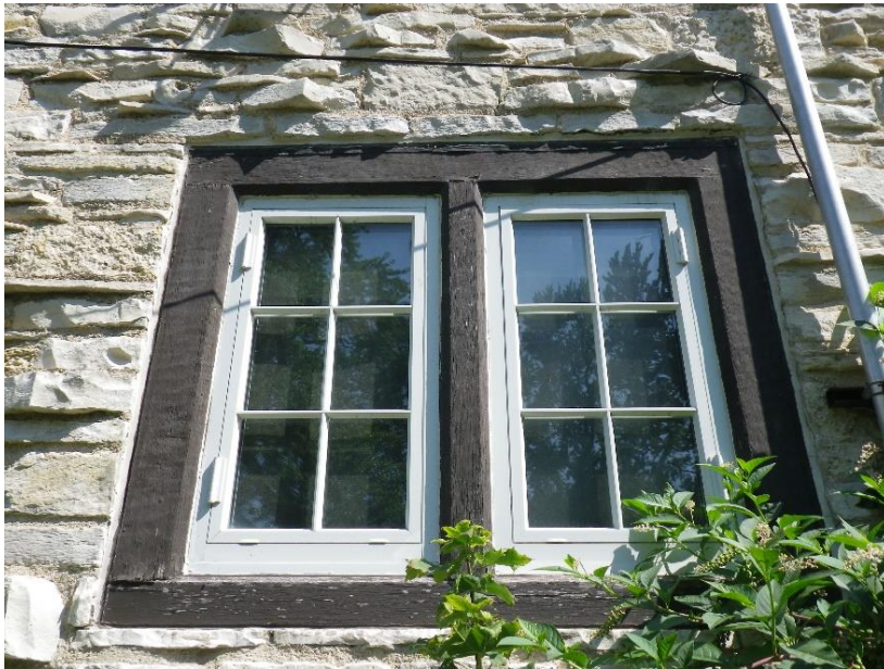
Figure 52. View of window on coach house (2016)
