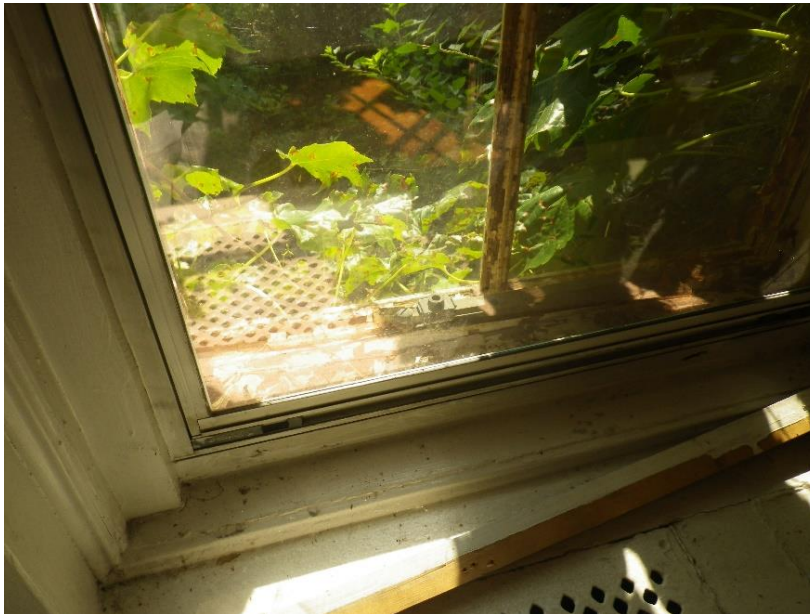
Figure 44. Non-historic interior storm window (2016)
