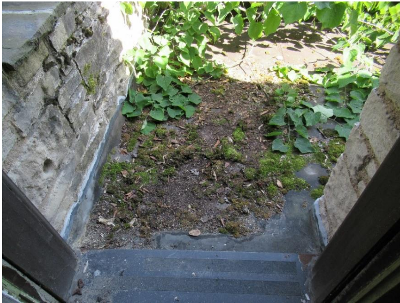
Figure 60. Coach house balcony
