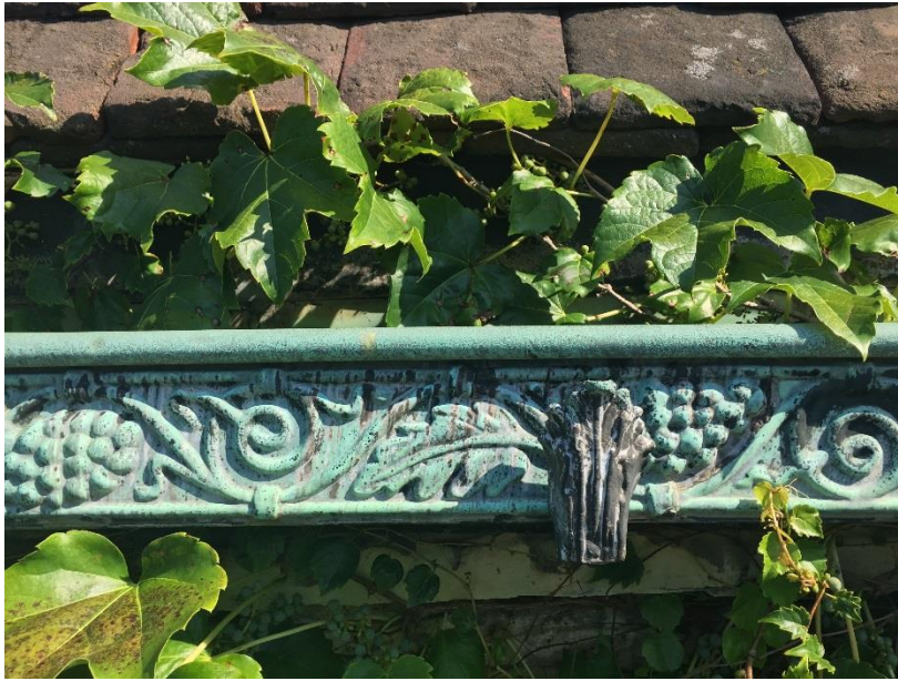
Figure 37. Vines growing in the gutter (2016)
