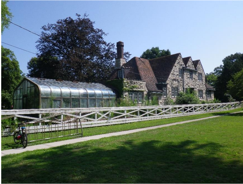
Figure 15. South facade and greenhouse at coach house (2016)
