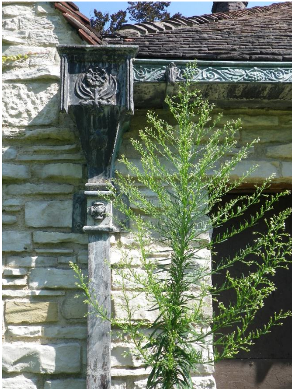
Figure 54. Conductor and downspout on coach house (2016)
