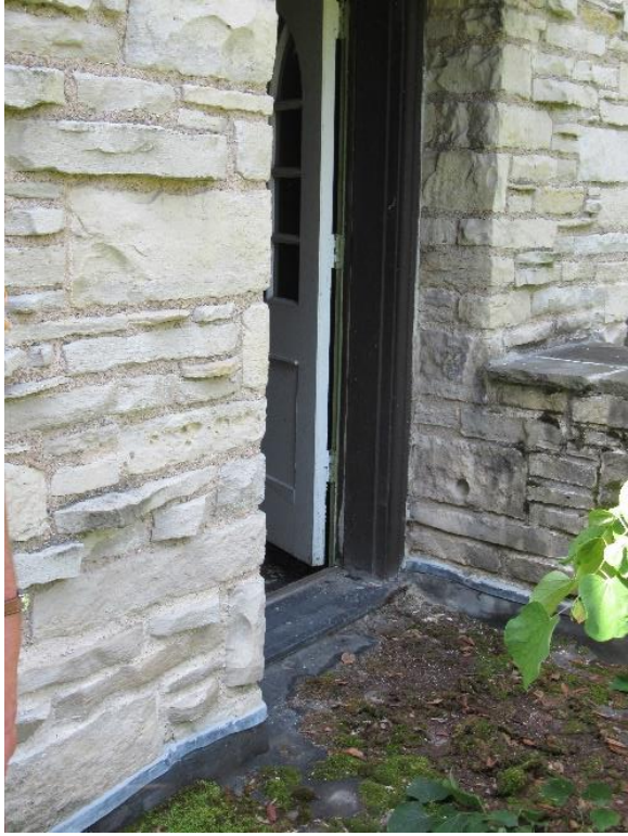
Figure 61. Coach house balcony
