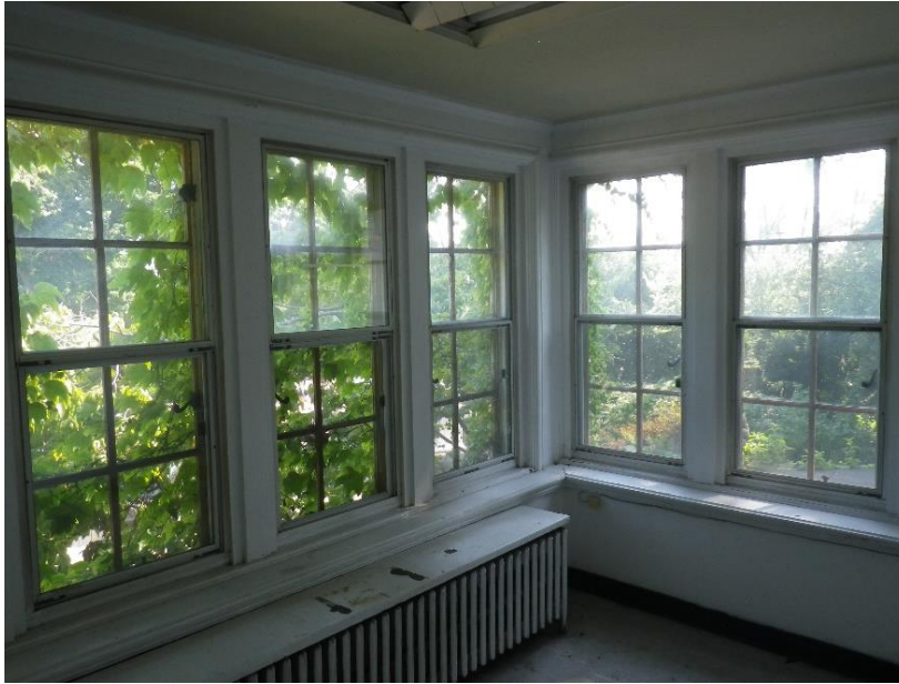
Figure 43. Steel windows with storm windows installed on interior (2016)
