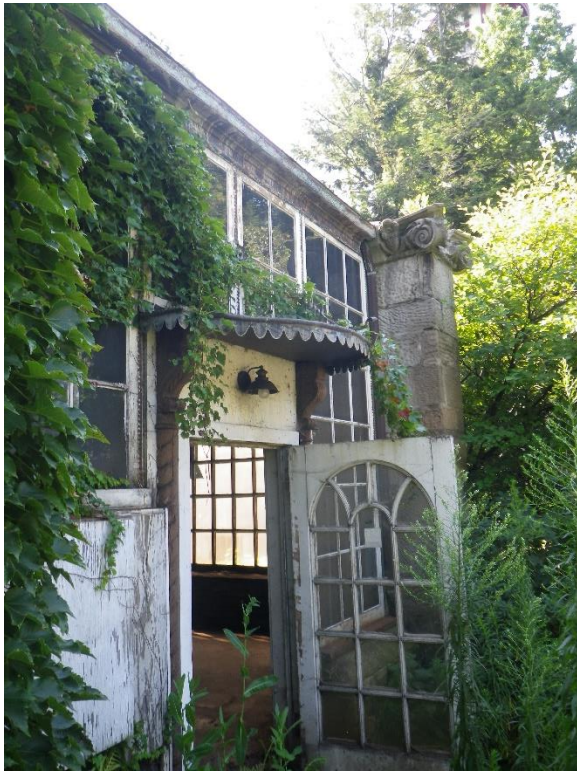
Figure 26. West facade of conservatory (2016)
