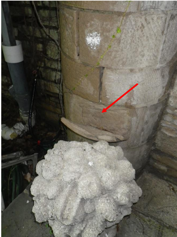
Figure 27. Spalling limestone (2016)
