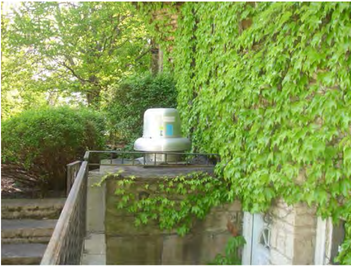
Basement photo area exhaust
