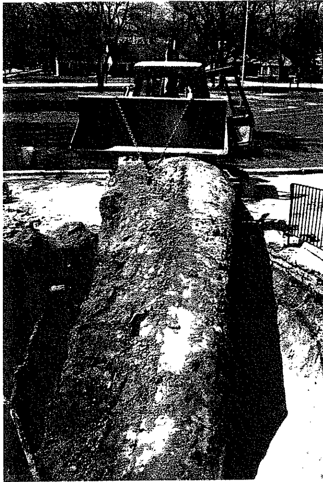
Photograph 3 Removing UST from Excavation Zone Direction of Photo: West
