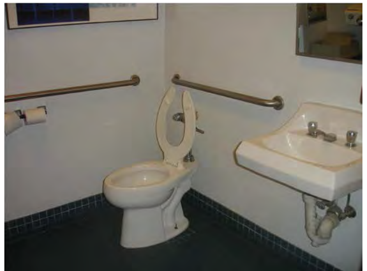
First floor handicapped toilet
