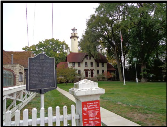
SOUTH ADJACENT PROPERTY (GROSS POINT LIGHTHOUSE)
