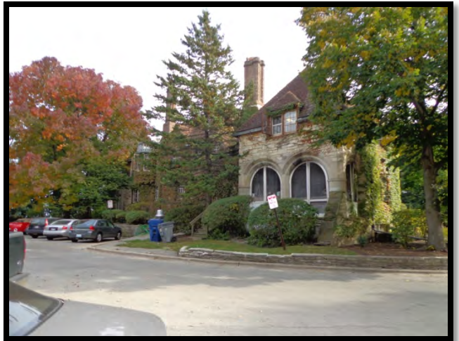
NORTH SIDE OF THE MAIN BUILDING
