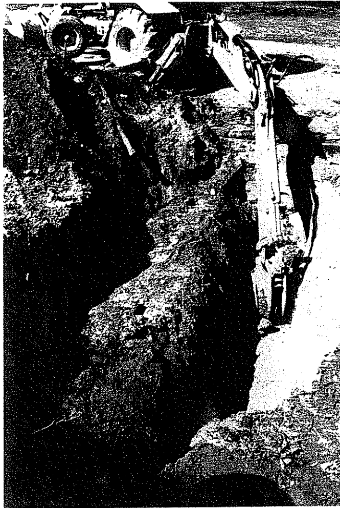
Photograph 1 Preparing Excavation Zone for UST Removal Direction of Photo: West
