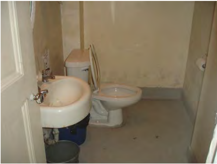
Basement toilet room
