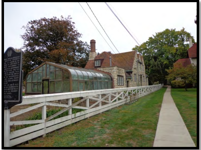
WEST & SOUTH SIDES OF THE COACH HOUSE
