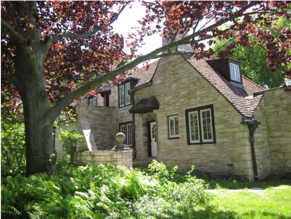
Photo 9. North Elevation of Coach House.
