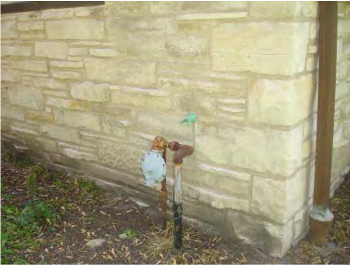
Gas service to coach house
