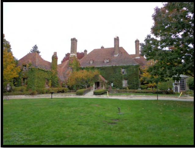
WEST SIDE OF THE MAIN BUILDING
