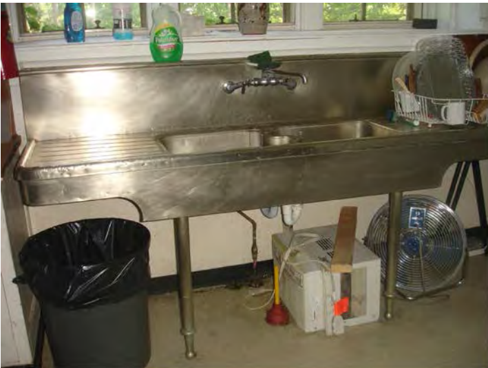
Sink in kitchen
