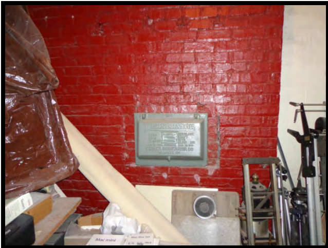
FORMER INCINERATOR IN THE BASEMENT OF THE MAIN BUILDING
