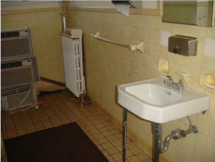
3rd floor toilet room
