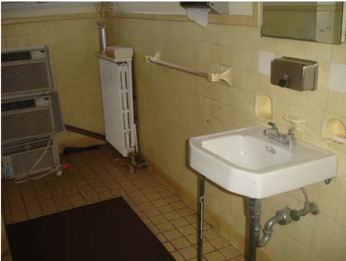
3rd floor toilet room
