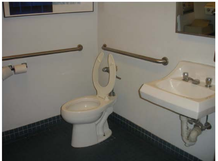
First floor handicapped toilet
