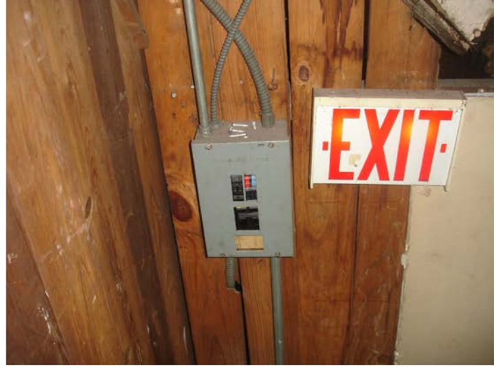
Panel at base of attic stairs
