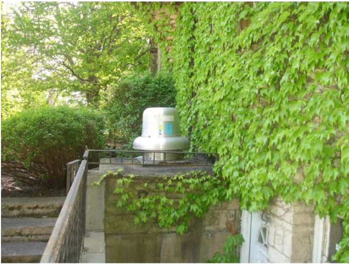
Basement photo area exhaust
