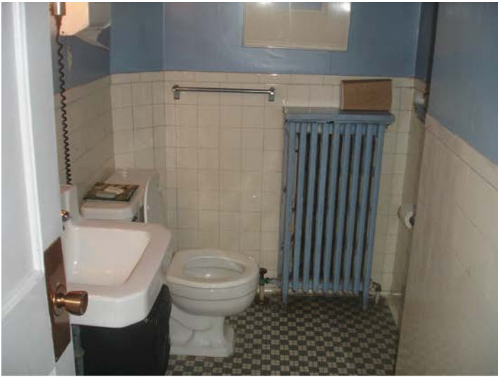
First floor toilet room
