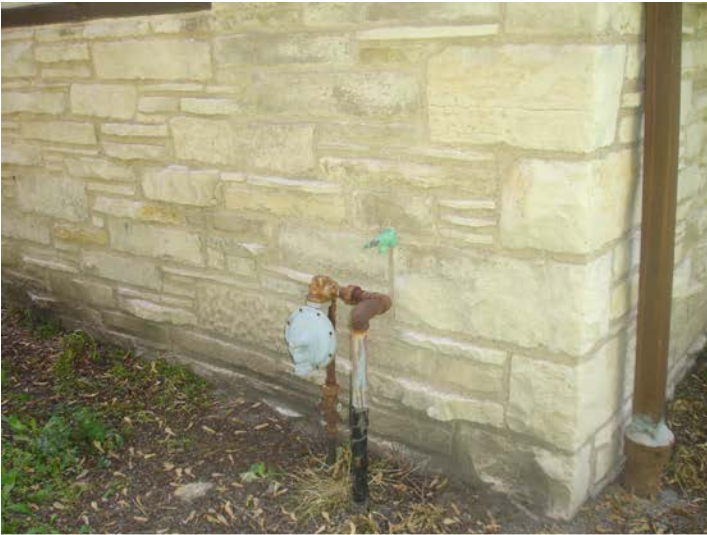
Gas service to coach house
