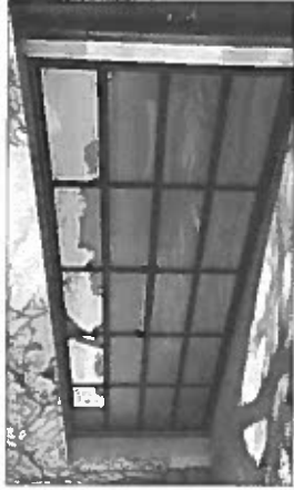
Frosted Glass Garage Door (at Parking & Loading entries):
