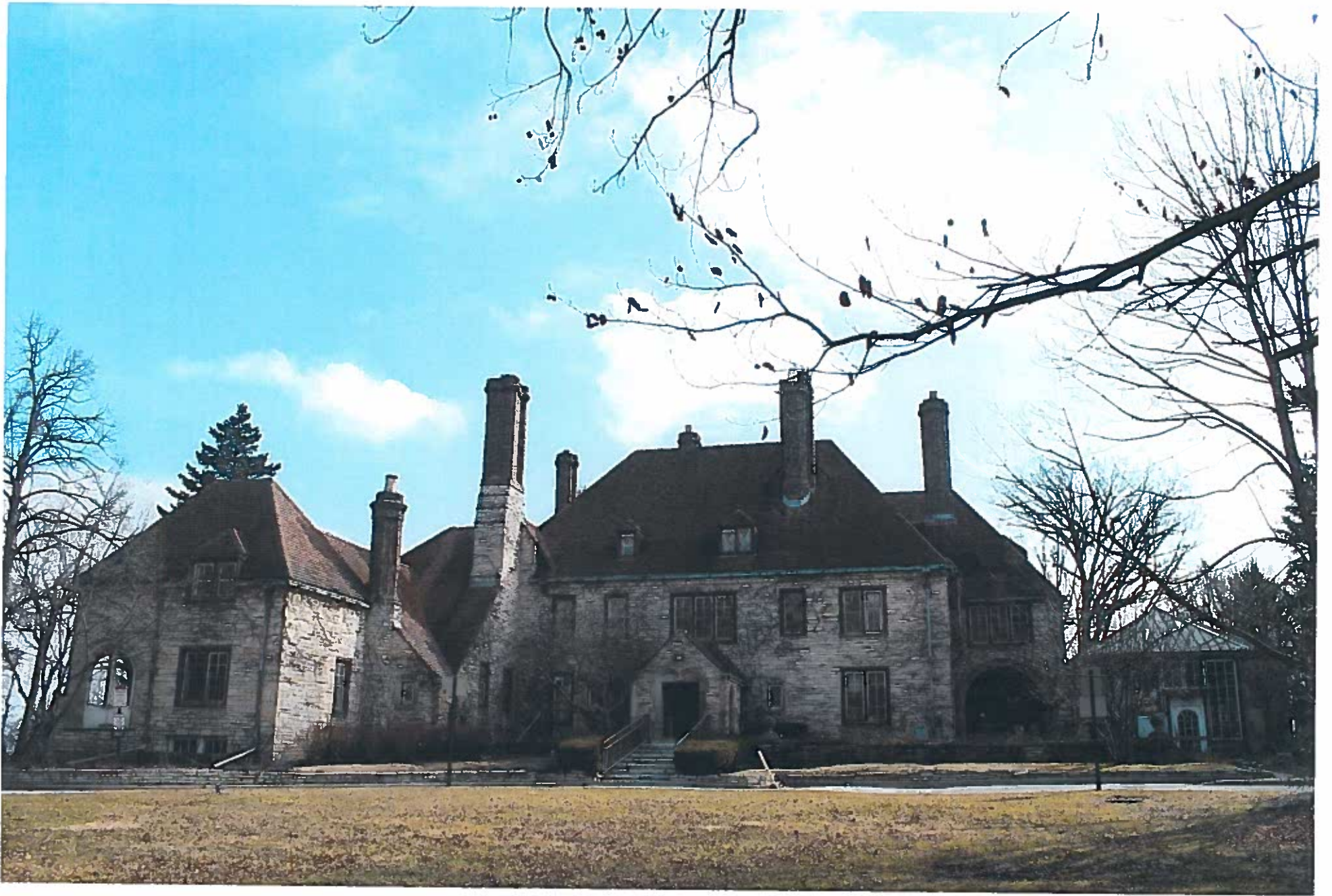
Existing - From Sheridan Rd.
