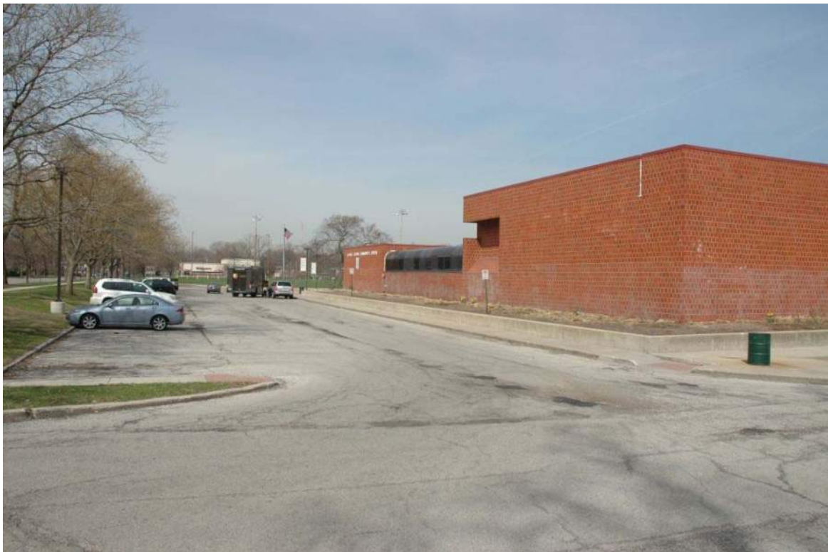
South Façade of Building as viewed from the Southeast
