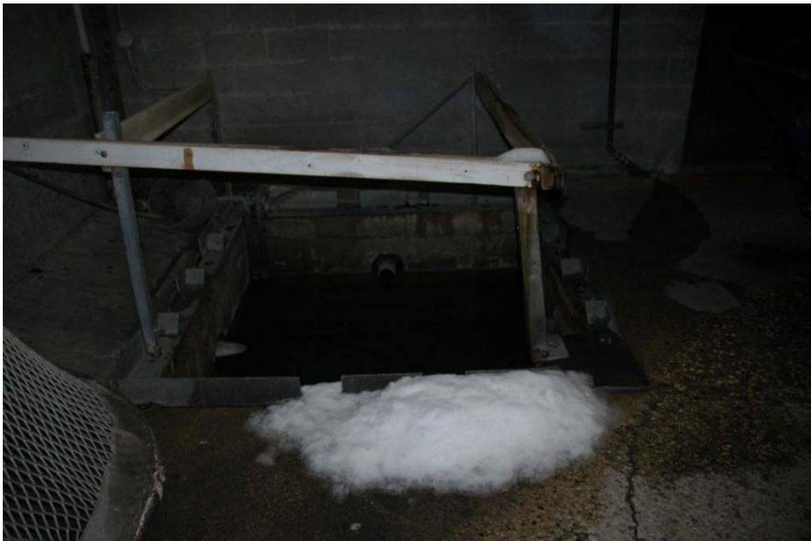
Pit within the Zamboni Room
