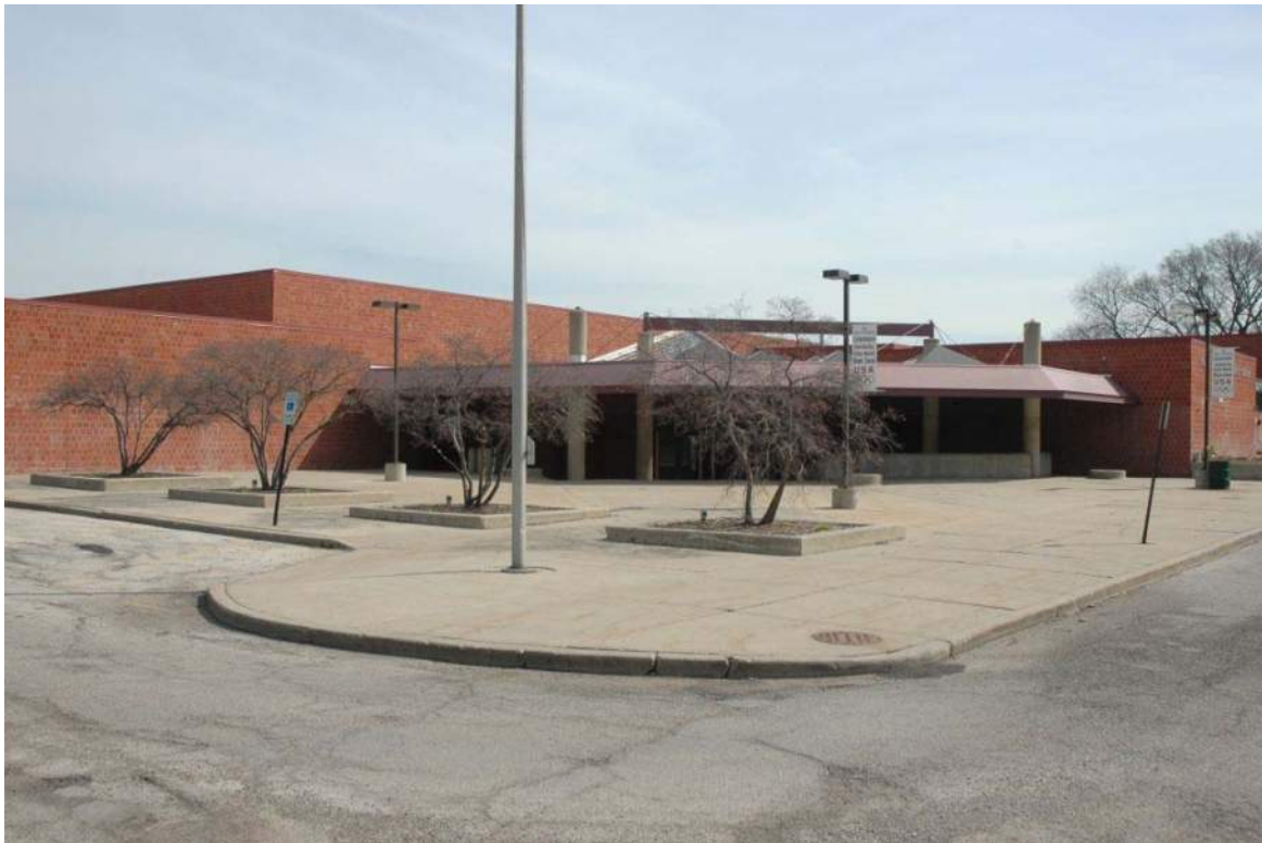
Subject Property Building as viewed from the Southwest
