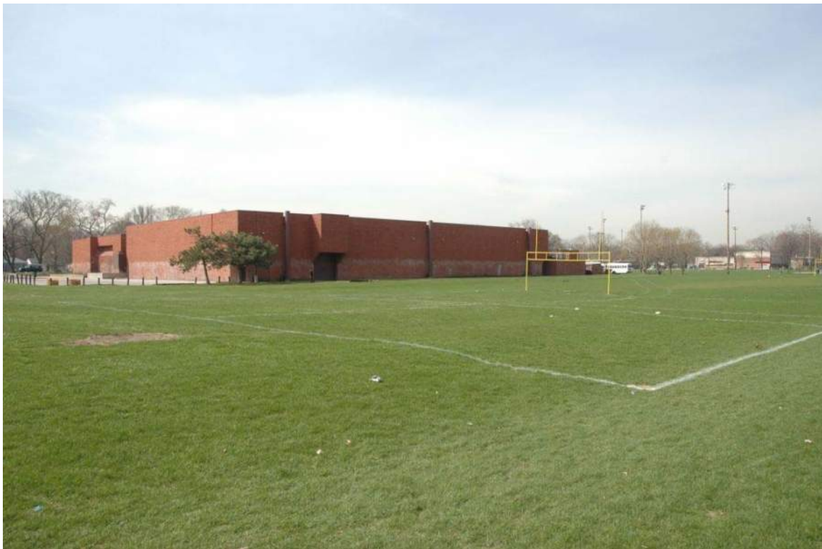
Subject Property as viewed from the Northeast Corner of the Site
