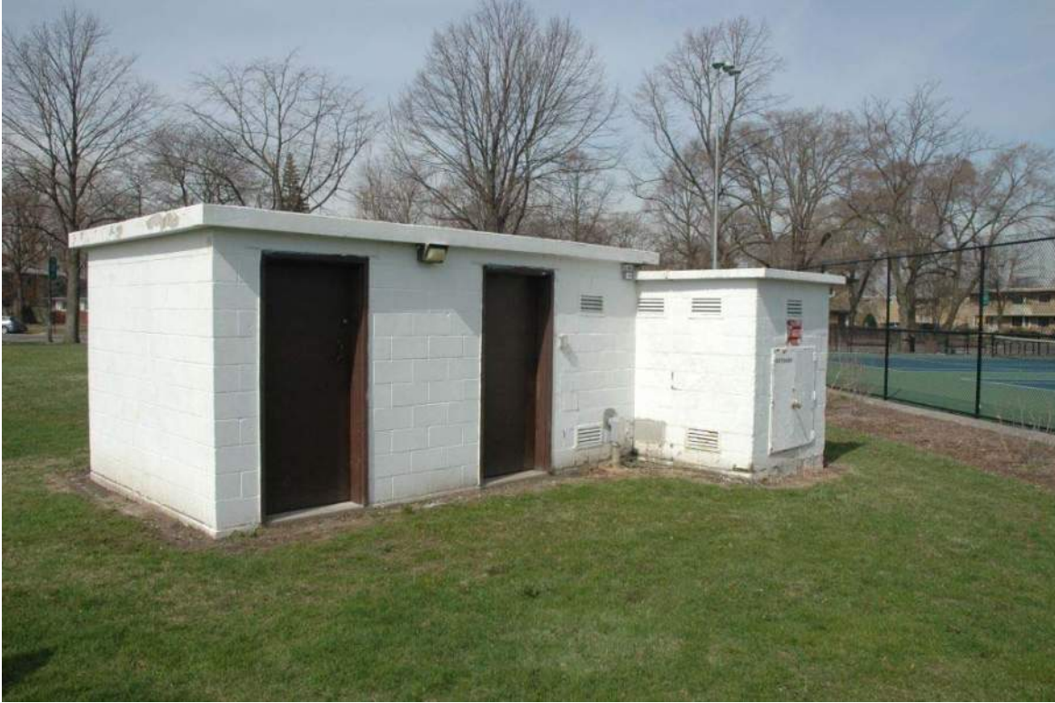
Lighting House/Electrical Vault Building Located at the Northwest Corner of the Site
