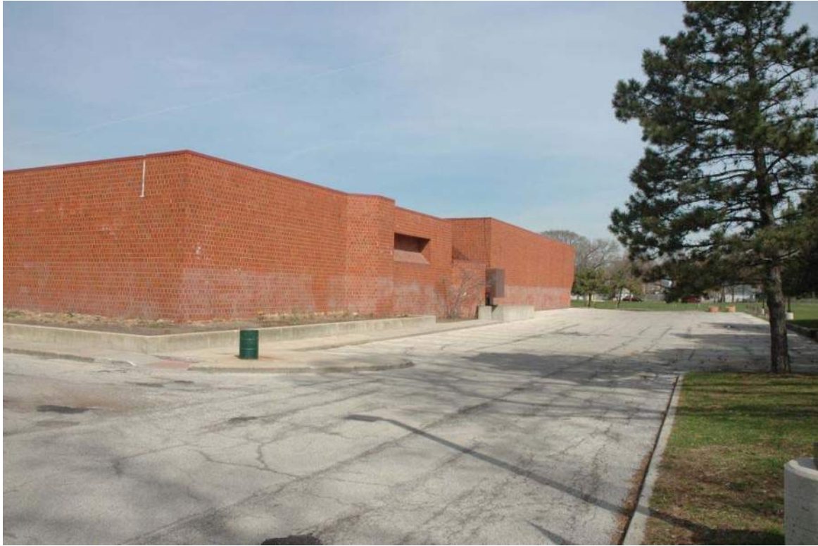
East Façade of Building as viewed from the South
