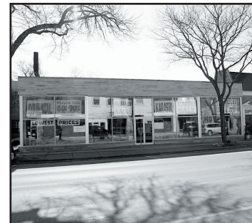
Some storefronts near Lincolnwood clutter windows with excessive signage.
