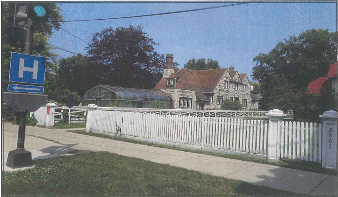
CARRIAGE HOUSE - WESTERN ELEVATION
