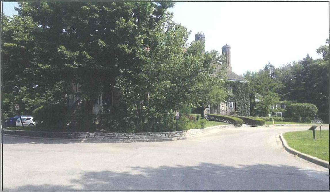
MANSION - FRONT, WESTERN ELEVATION
