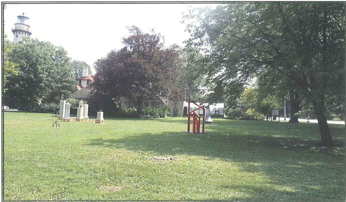
CARRIAGE HOUSE - NORTHERN ELEVATION
