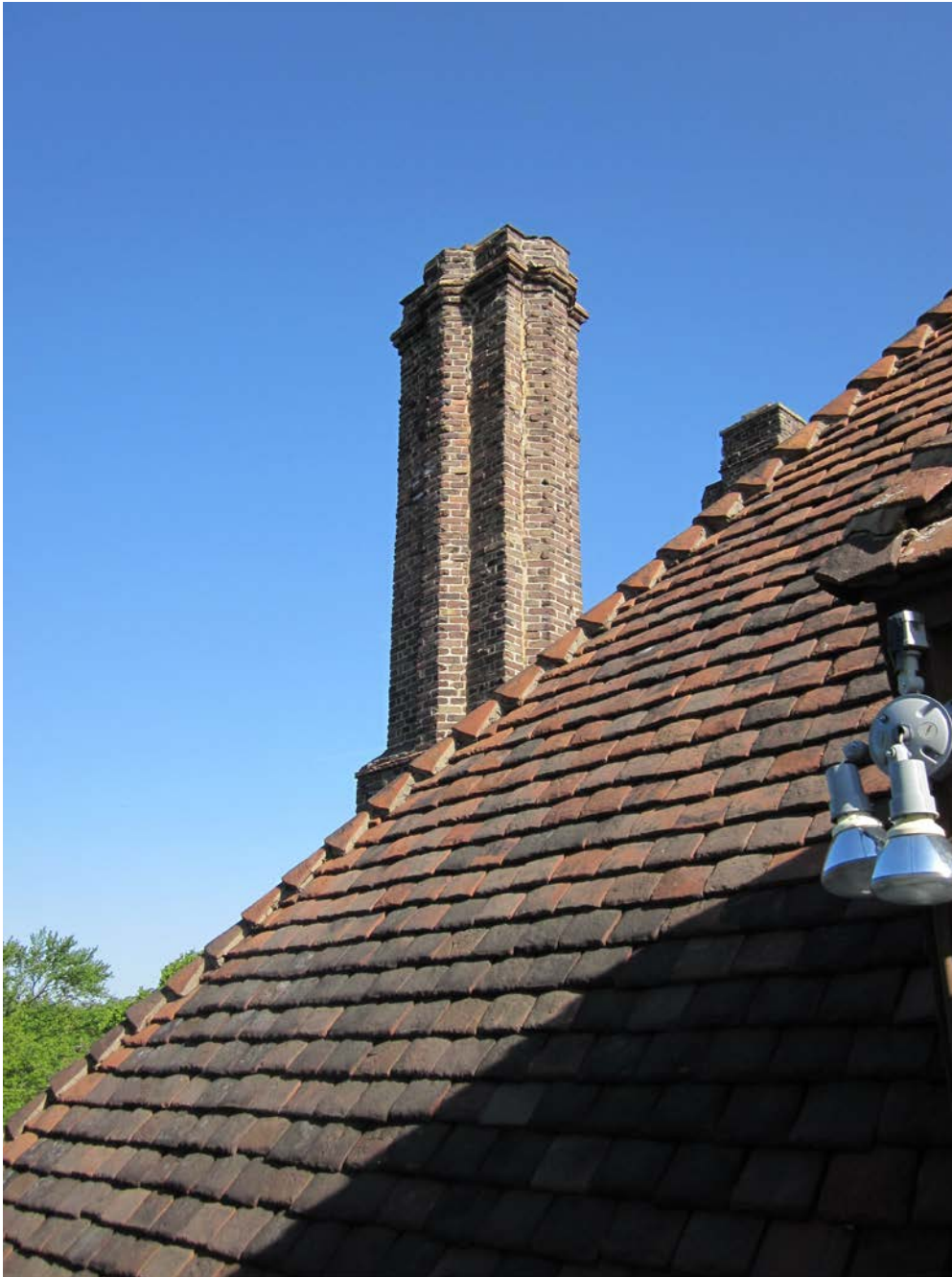
Photo 7 – View of roof tiles and chimney, south elevation.
