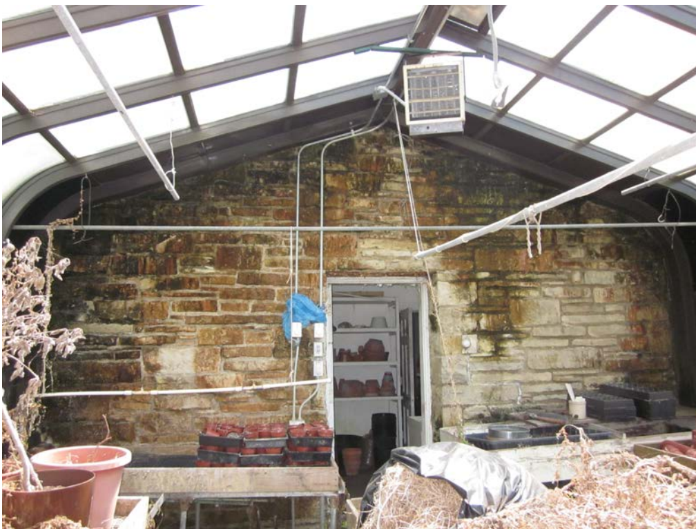
Photo 10. Interior of greenhouse, looking east.
