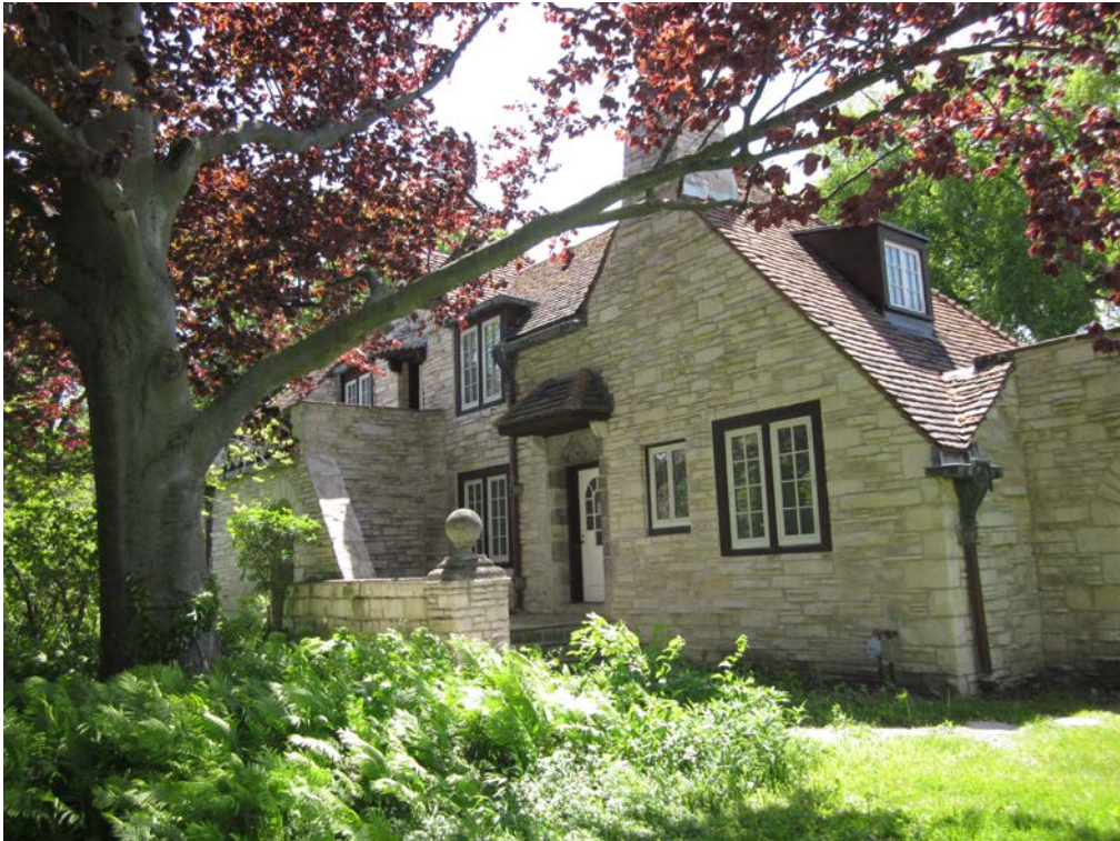
Photo 9. North Elevation of Coach House.
