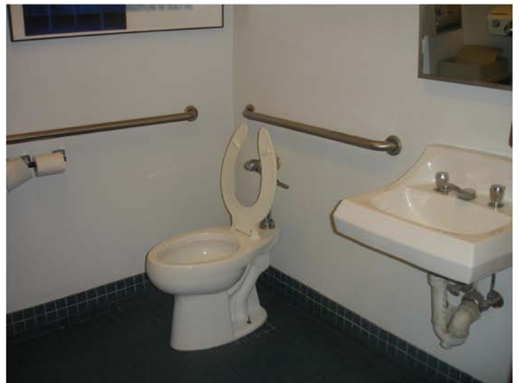
First floor handicapped toilet
