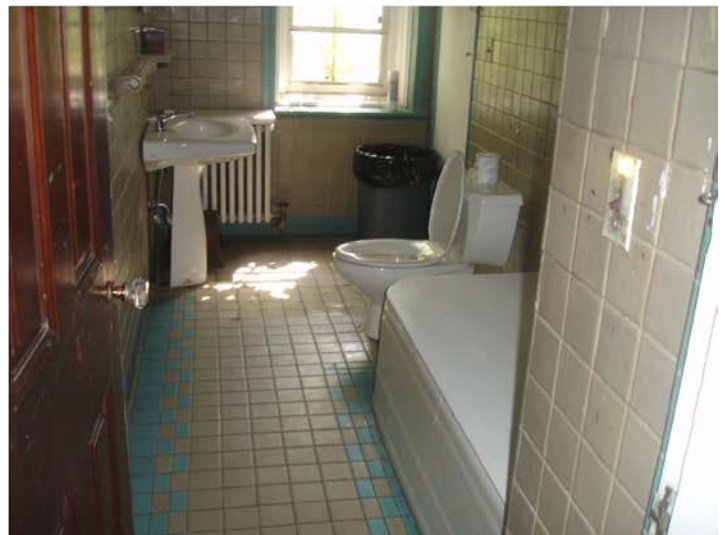
2nd floor toilet room
