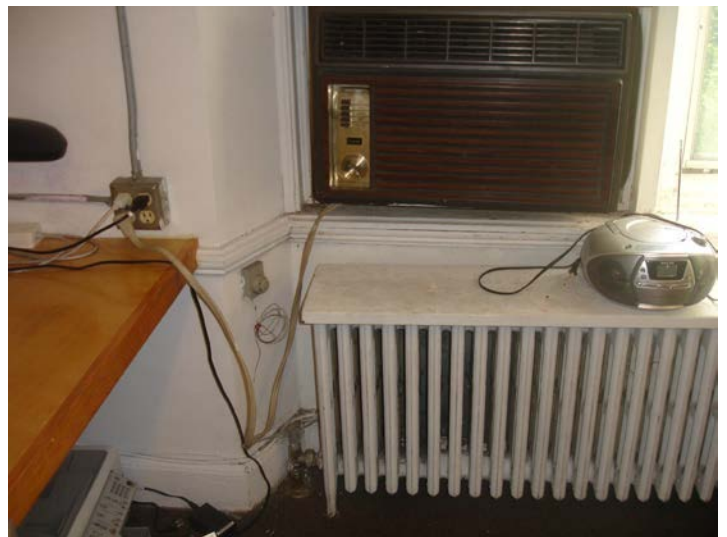
3rd floor office
