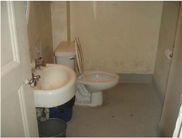
Basement toilet room
