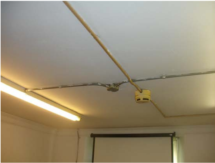
Ceiling of 3rd floor office
