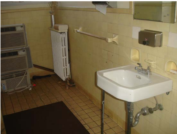
3rd floor toilet room
