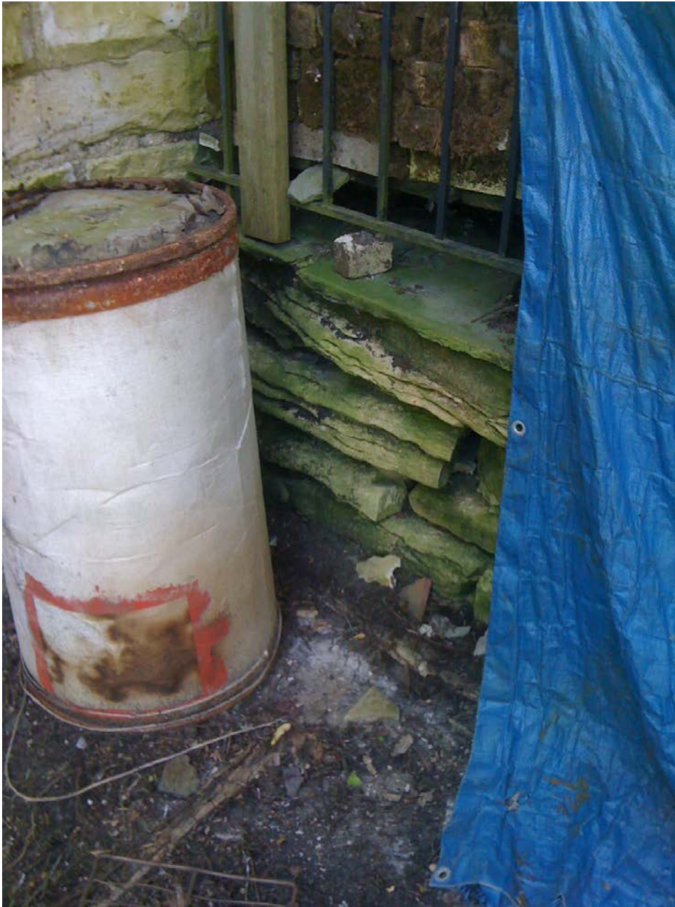
Photo 4 – Masonry at original north stair.
