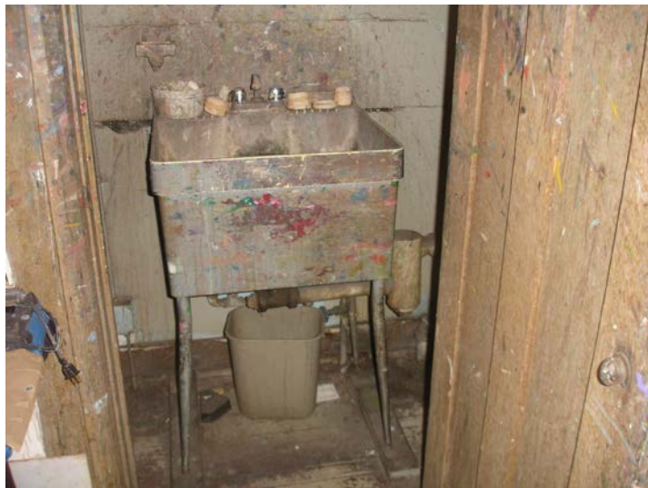
Slop sink in 3rd floor art studio
