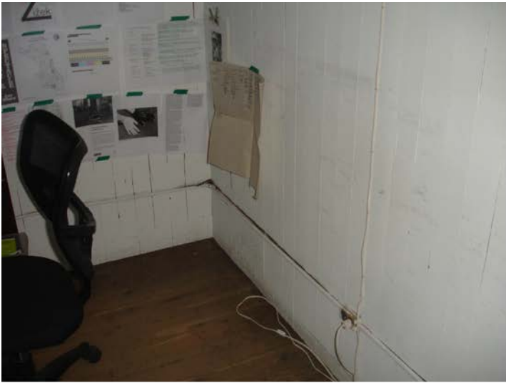
3rd floor office
