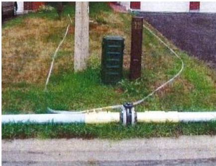
Temporary water main with hose connections to two houses
