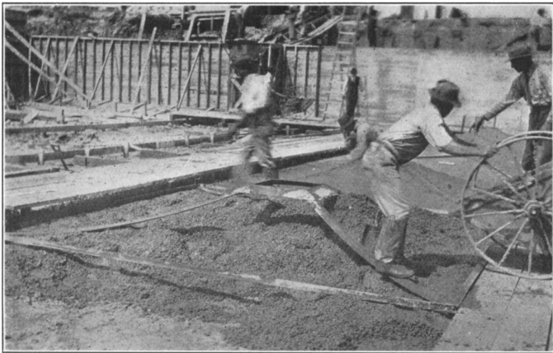
FIG. 6. STEEL SCREED FOR INVERTED GROINED ARCHES
