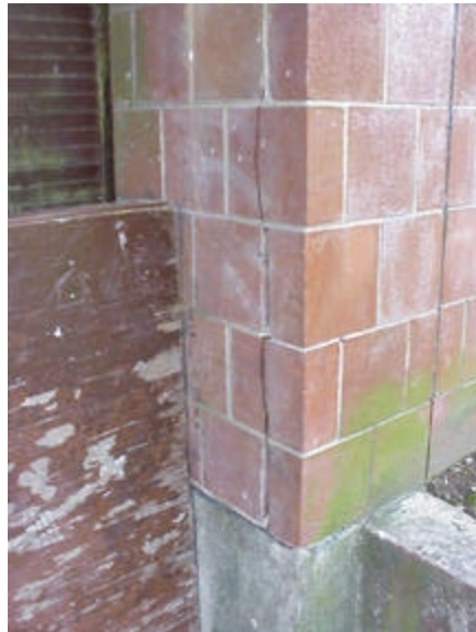
Photo A-9: West Overhead Door Jamb
