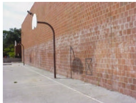
Photo A-6: East Wall - Overall
