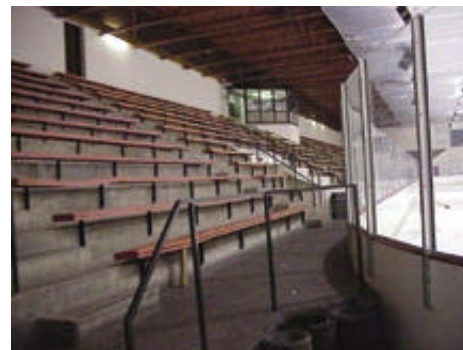
Photo A-14: Ice Rink/Bleachers Showing Sound Booth
