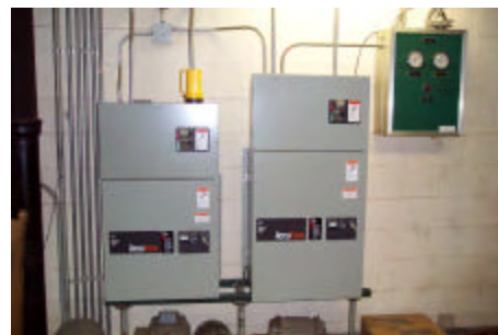
Photo E-2: Variable Frequency Drives in Rooftop Mechanical Room
