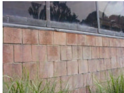
Photo A-5: South Wall Sill Detail
