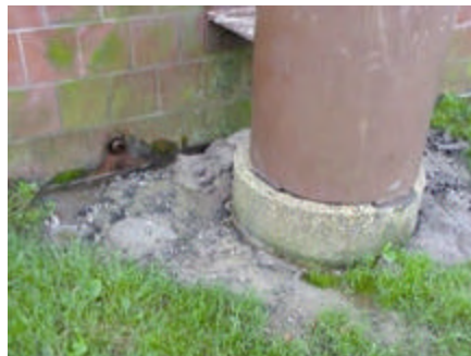
Photo A-8: North – Downspout Detail
