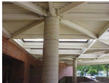
Photo A-17: Main Canopy
