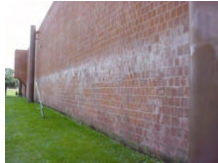
Photo A-2: North Side Masonry Wall – Showing Graffiti Block
