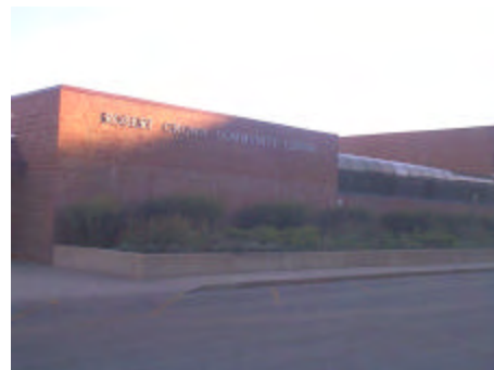
Photo O2: Main Street façade of the Robert Crown Center
