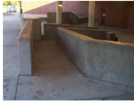
Photo HC-1: Existing Handicap Ramp
