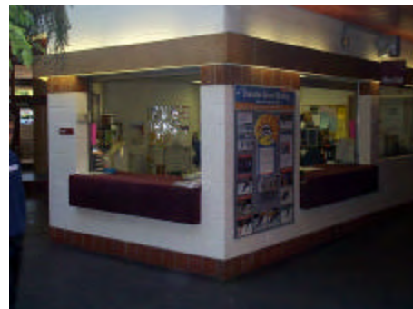
Photo HC-6: Non-compliant Building Reception Counter
