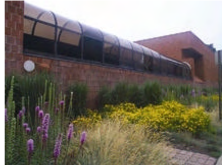
Photo A-4: South Wall Skylight
