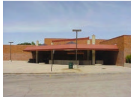
Photo A-1: Overall Front Entry
