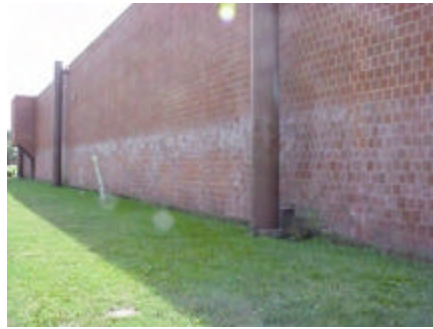
Photo A-7: North – Overall Elevation
