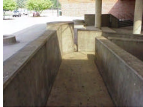
Photo A-18: Main Entry Ramp
