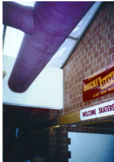
Photo R-2: View of leakage area at the northwest corner of the main skylight.
