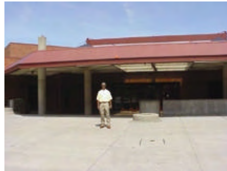
Photo A-16: Main Entry
