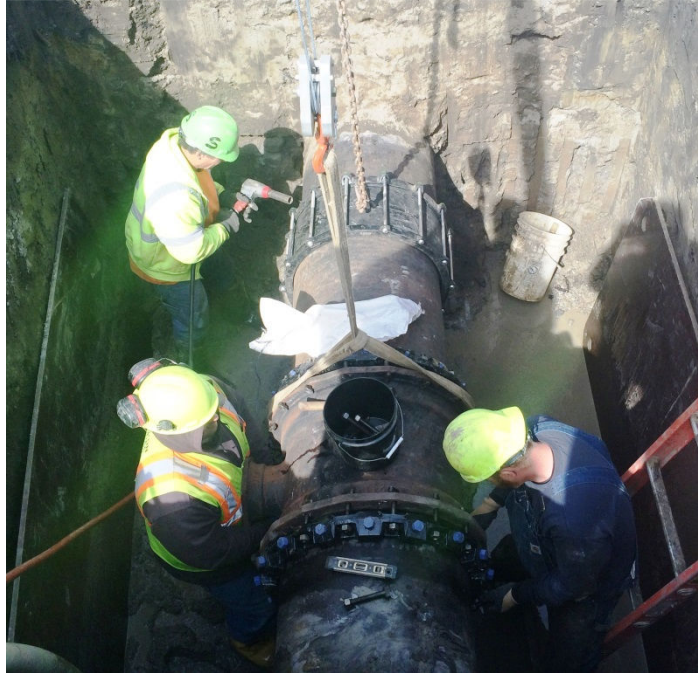
A Distribution Division field crew installing a new fire hydrant connection on a 24" diameter water main, to improve the City's ability to clean and test this main.
