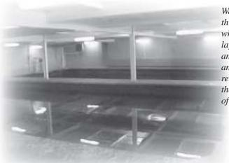
Water flows through filters which contain a layer of anthracite coal and filter sand, removing the tiniest of particles.
