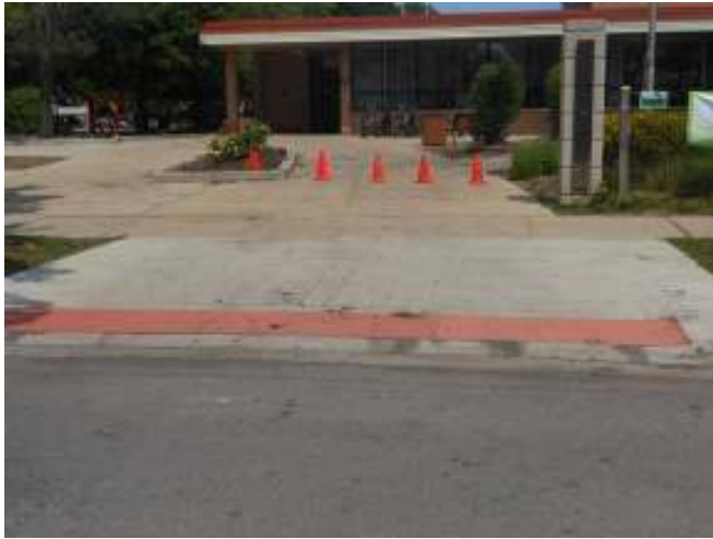
Depressed curb at Foster Street for south entrance drop-off
