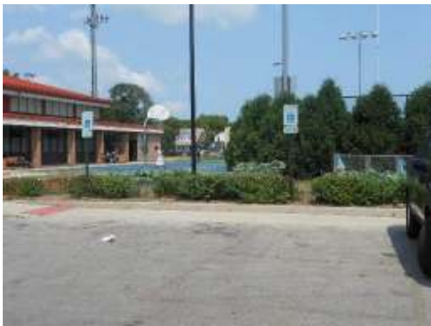
Two accessible parking spaces and a curb ramp to access Fleetwood
