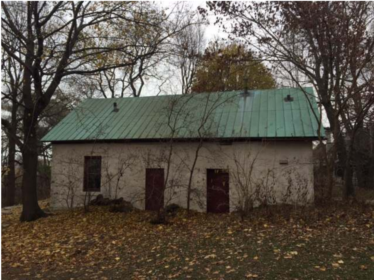
North Fog House with Existing Standing Seam Copper Roof
