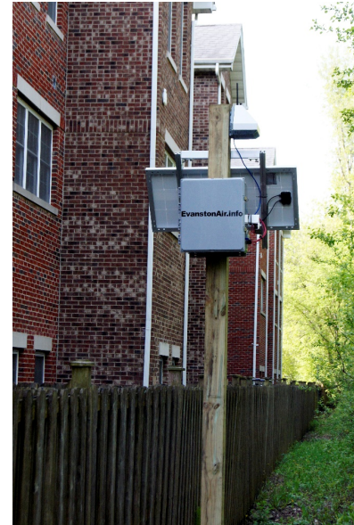
Figure 5: Station 3 at Church St. Village – East side of waste transfer station.
