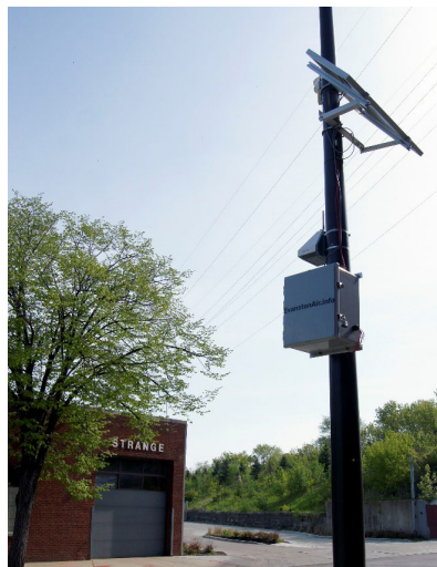
Figure 6: Station 4 at 1715 Church St. along south side of waste transfer station.
