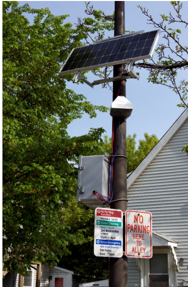
Figure 3: Station 1 at 1721 Lyons St. – West side of waste transfer station.
