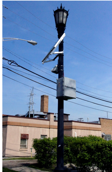
Figure 4: Station 2 at 1670 Lyons St. – Northeast side of waste transfer station.
