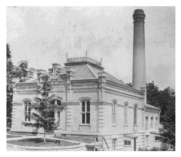
The original Water Works was built in 1874 to provide water for Evanston's 3,500 residents. The system consisted of a 16-inch intake pipe extending 1,200 feet into the lake, a small Holly steam engine capable of pumping 2 million gallons per day, a hand fired boiler, and a few miles of cast iron water main. The original cost of the steam engine and boiler was \$24,000. During the first year of operation the plant pumped 95 million gallons of water.
