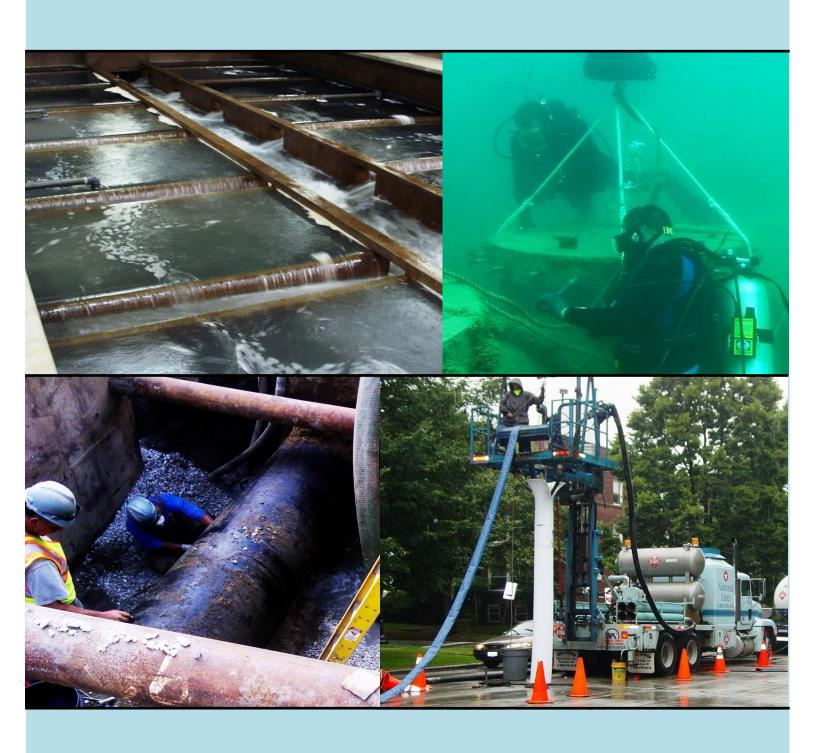
Cover photos, clockwise from top left: cleaning the filters at the Evanston Water Treatment Plant; Evanston Utilities Department divers inspecting one of the City's water intakes in Lake Michigan; installation of a cured-in-place pipe (CIPP) liner in a City sewer main to rehabilitate the pipe; and installation of a 24" diameter water main under Davis Street in conjunction with the 2013 Davis Street reconstruction project.
