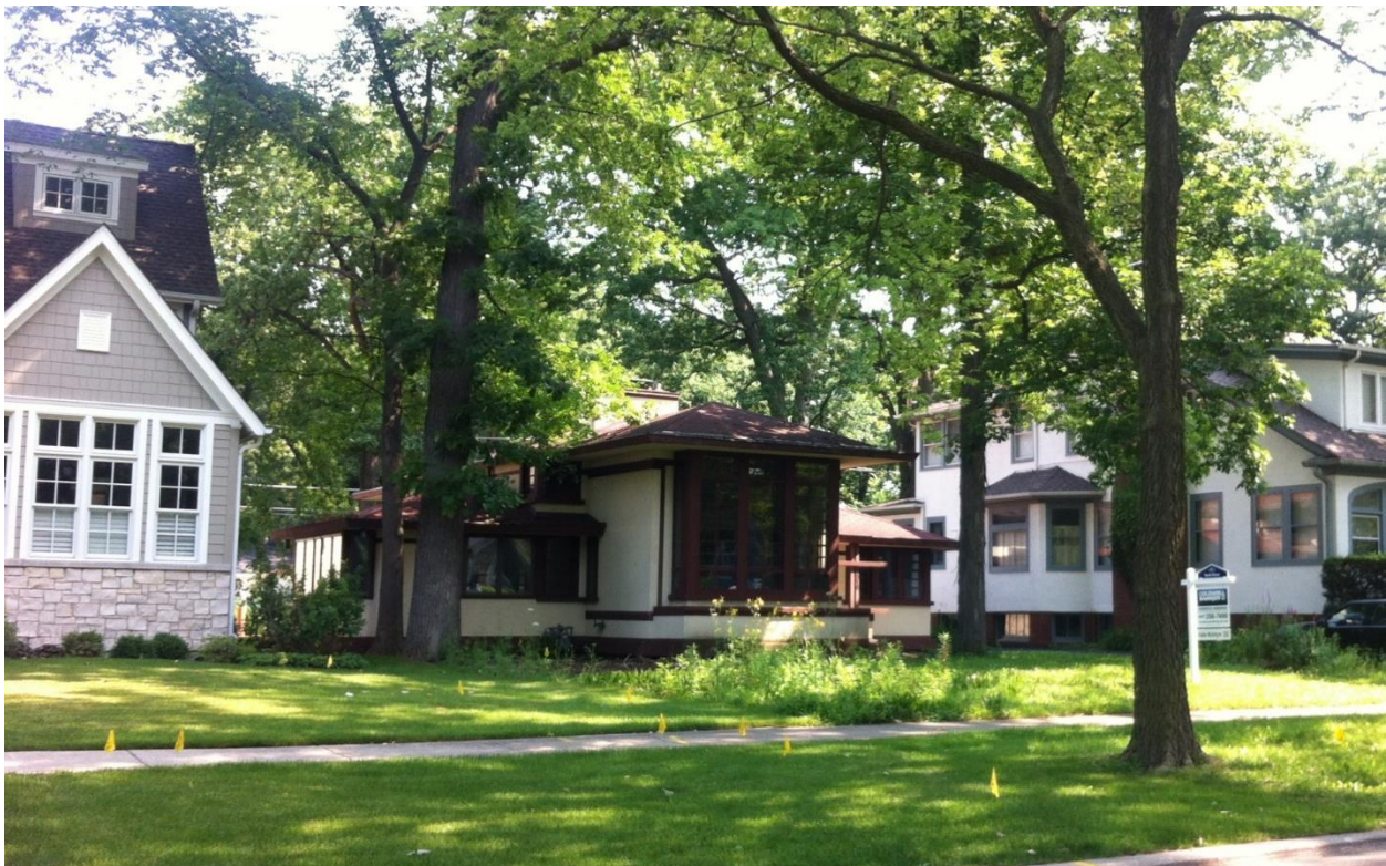
Photo 2: South façade at original Wilmette site.
