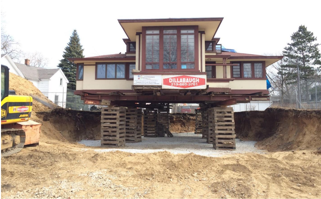
Photo 17: Raising of sections on new site.
