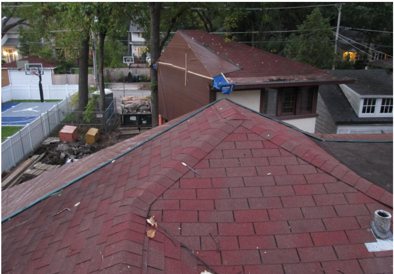
Photo 10: Moving of house sections on original Wilmette site.
