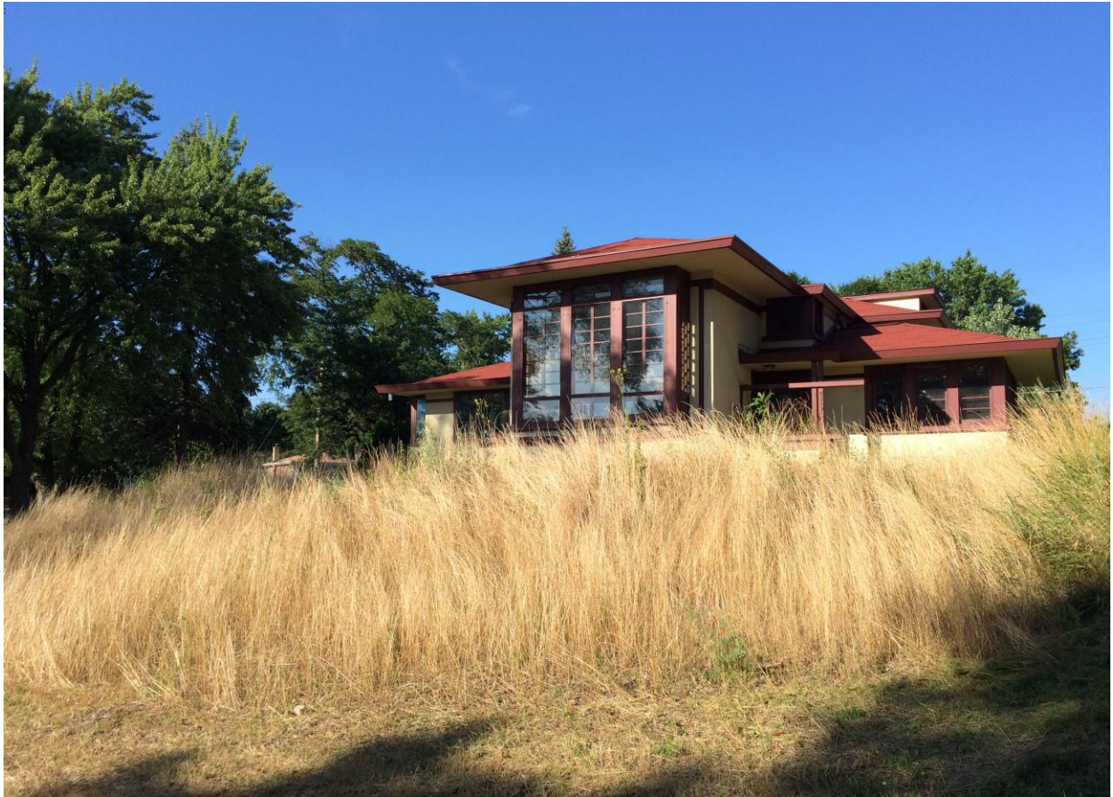
Photo 1: Current view of south façade.
