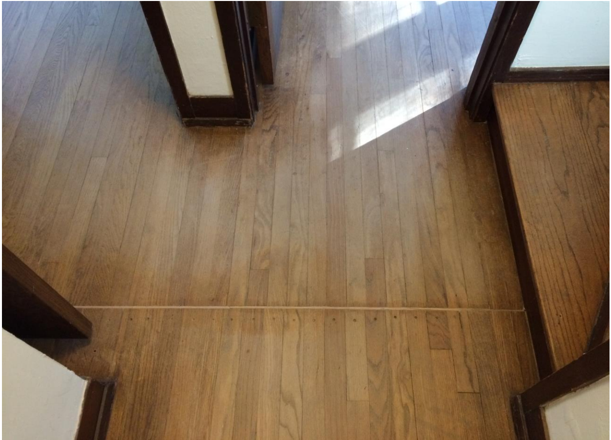
Photo 45: Upper level hallway view of repaired section cut line.
