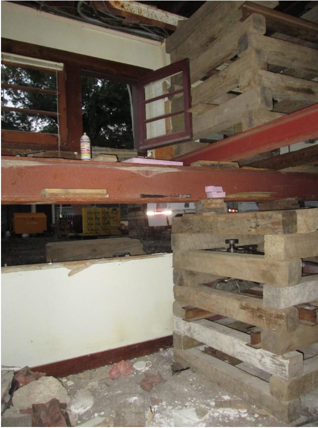
Photo 7: Process of raising rear section of house.
