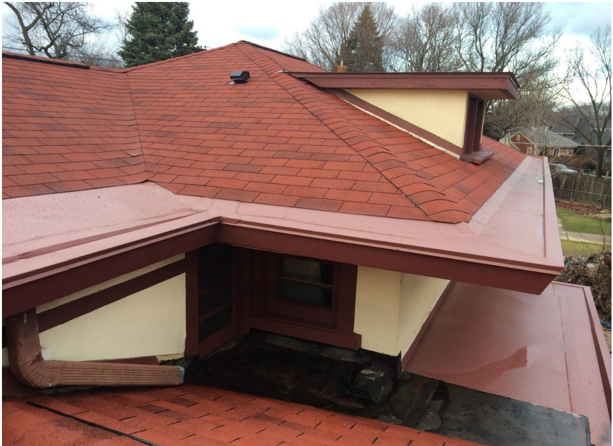
Photo 20: New roofing and restored built-in gutters.
