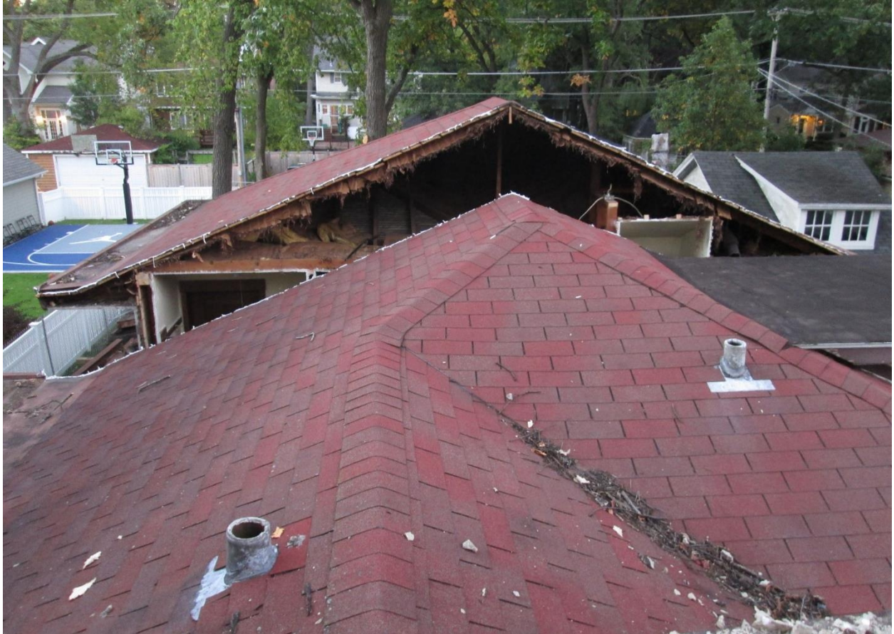
Photo 6: Process of raising rear section of house.
