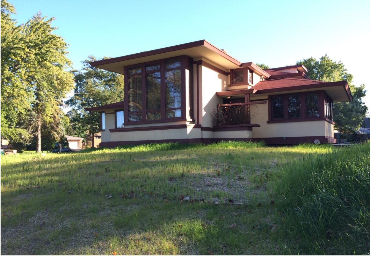
Photo 21: South façade at new site.
