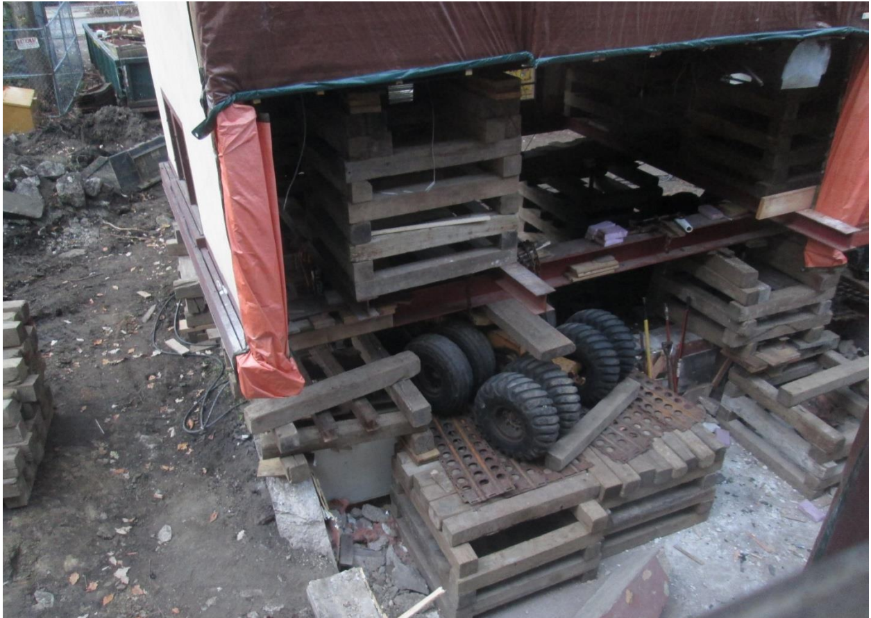
Photo 9: Moving of house sections on original Wilmette site.
