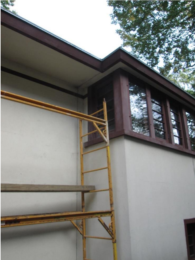
Photo 3: Process of cutting house.
