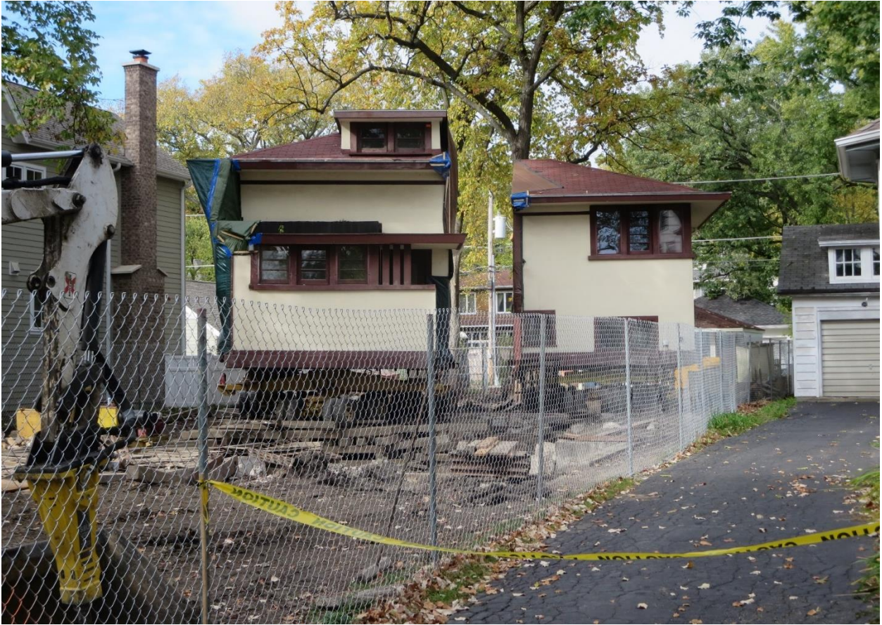
Photo 13: Moving of house sections on original Wilmette site.
