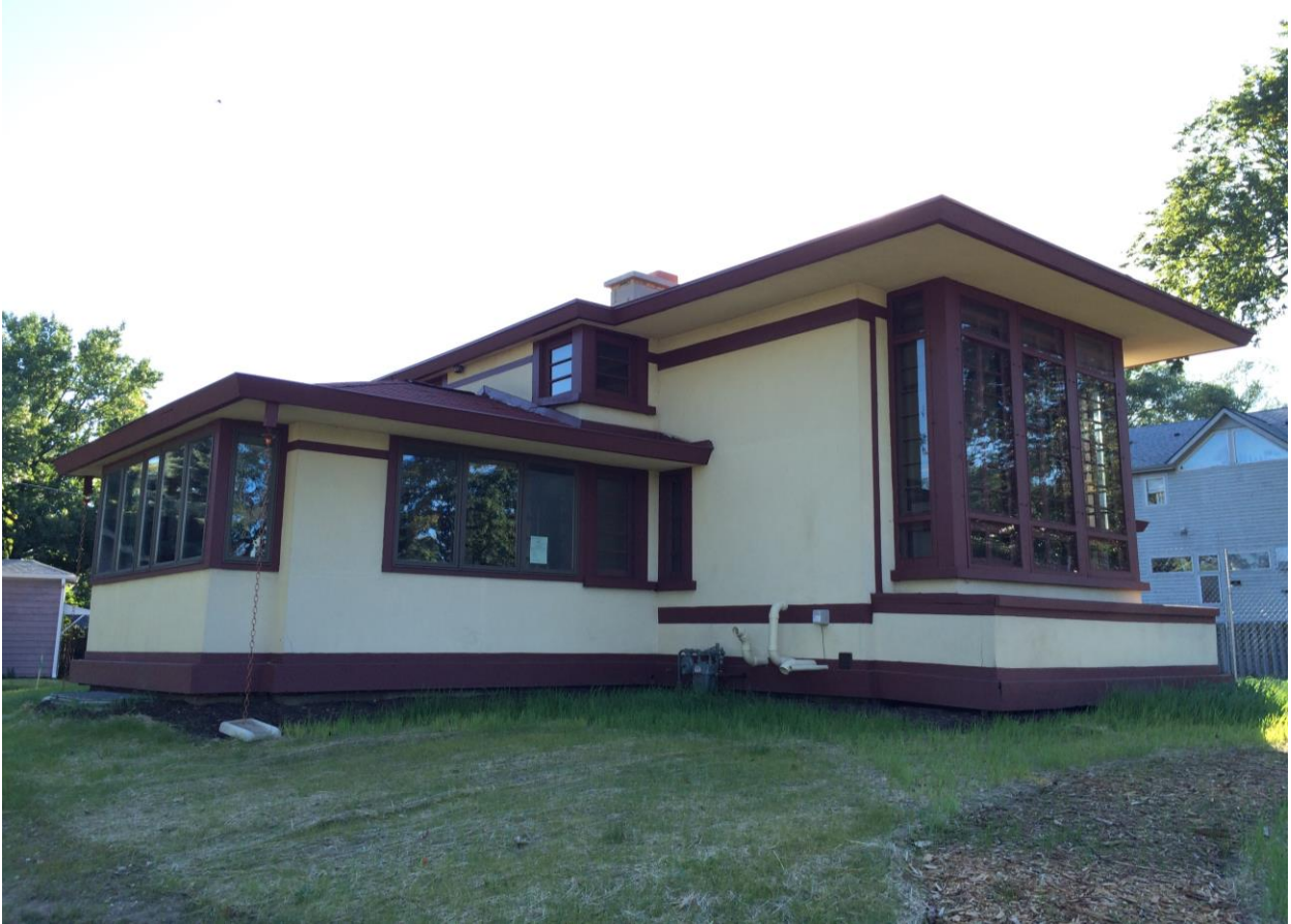
Photo 22: South façade, west end.
