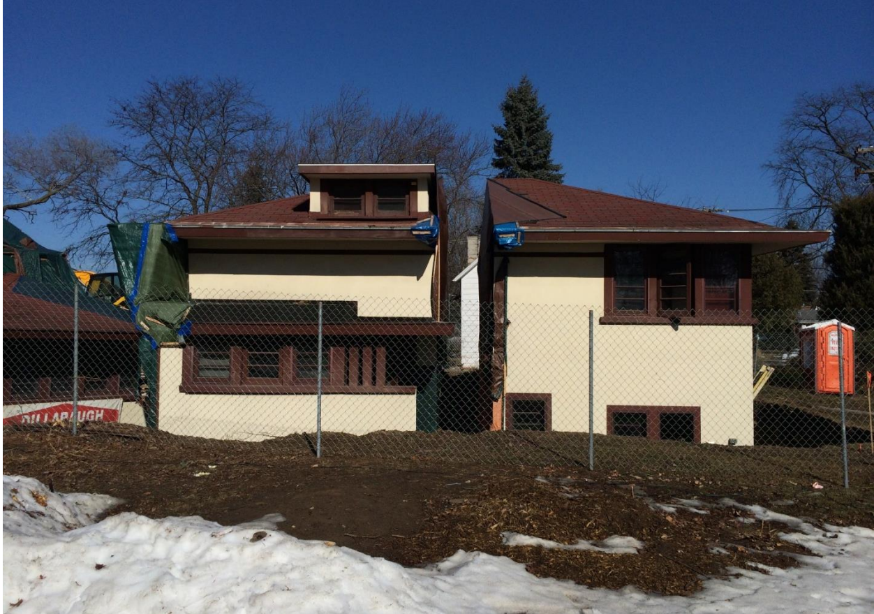
Photo 16: March 2015 positioning of sections on new site.
