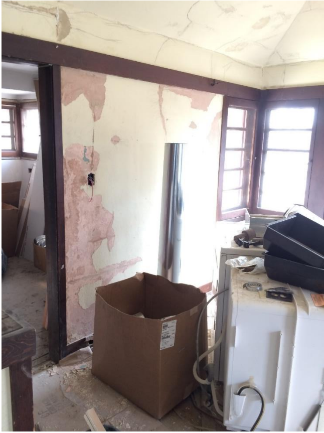
Photo 19: Typical interior repairs.
