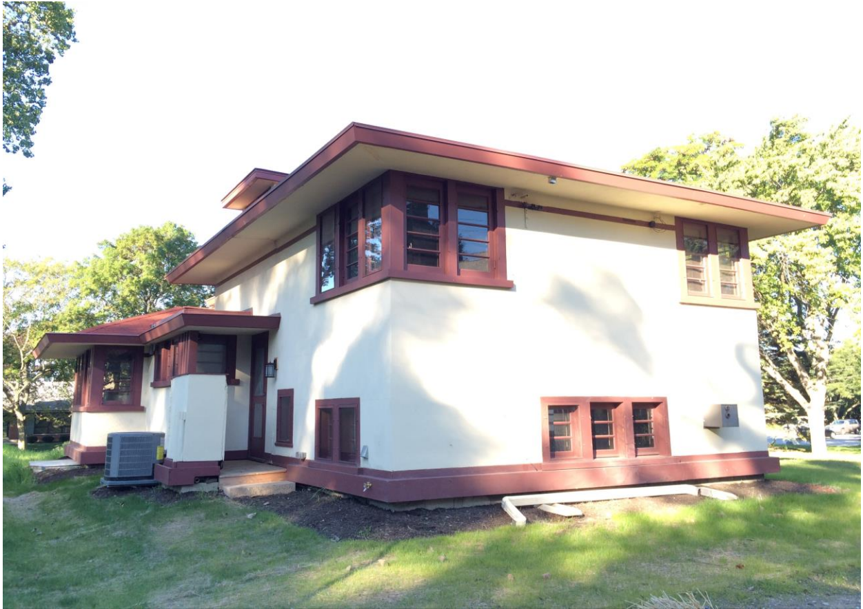
Photo 25: North and east facades.
