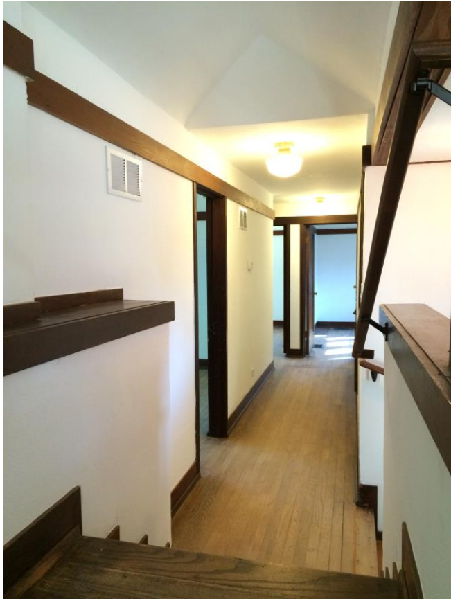
Photo 44: Upper level hallway viewed from loft.
