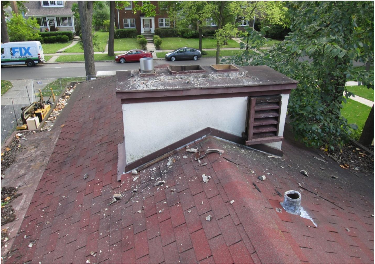
Photo 5: Chimney prior to removal.
