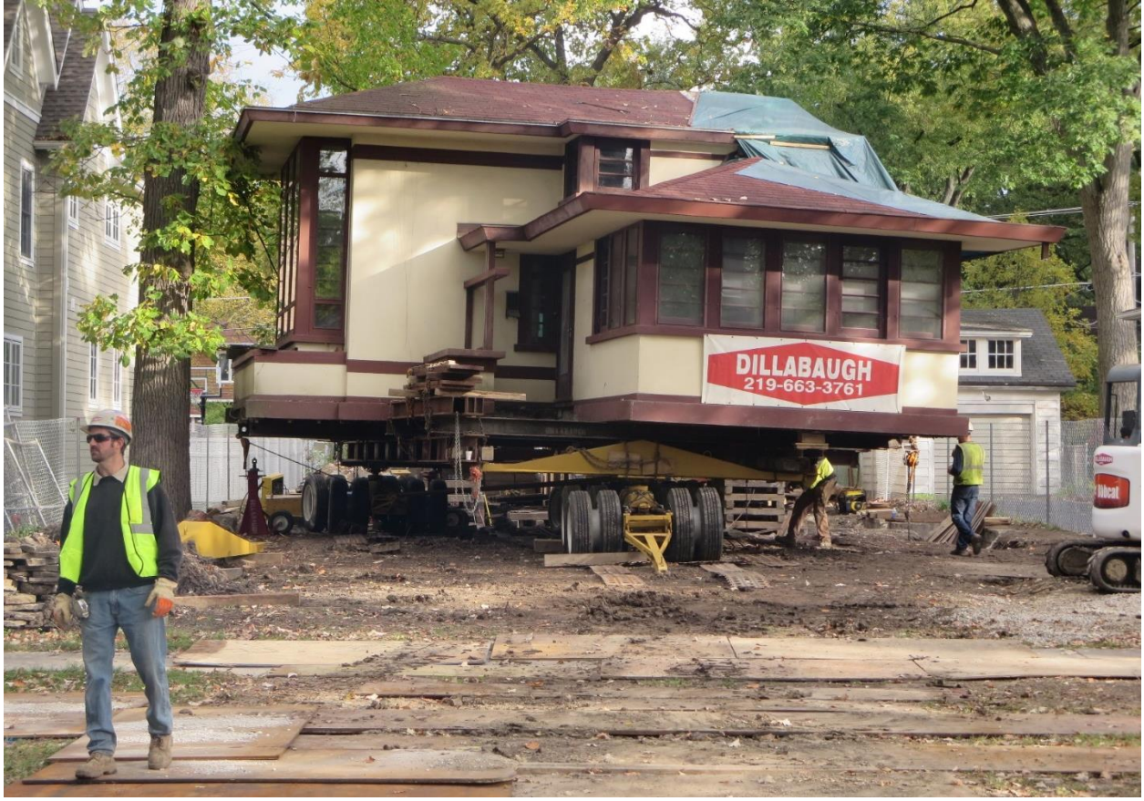
Photo 12: Moving of house sections on original Wilmette site.
