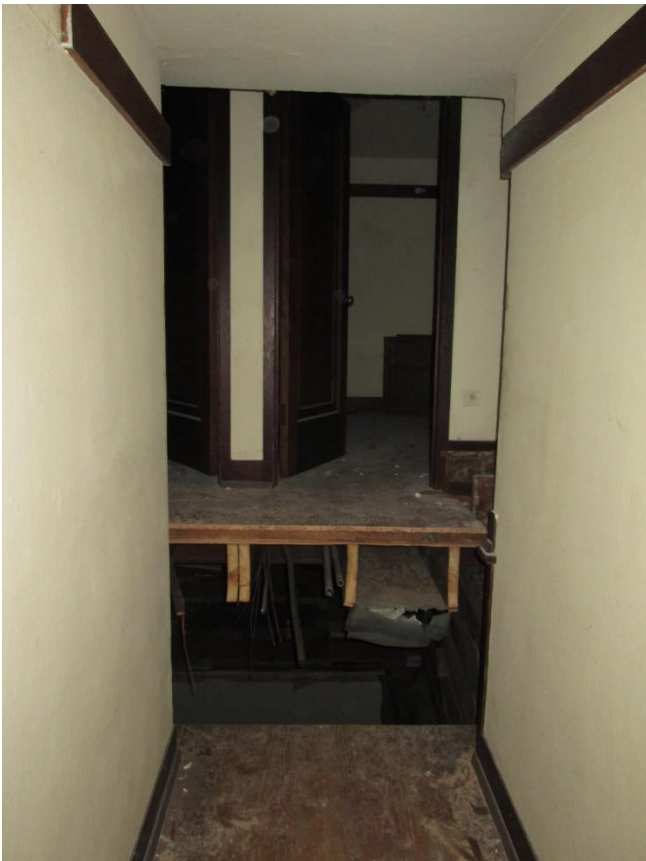
Photo 8: Process of raising rear section of house.
