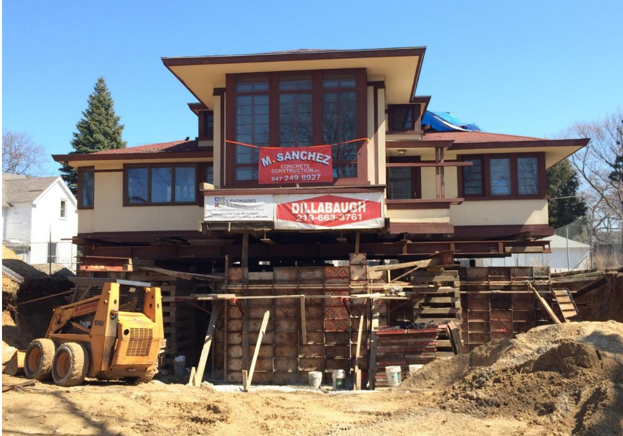
Photo 18: Pouring of new foundations below house sections.
