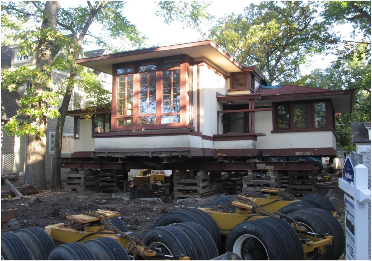
Photo 11: Moving of house sections on original Wilmette site.
