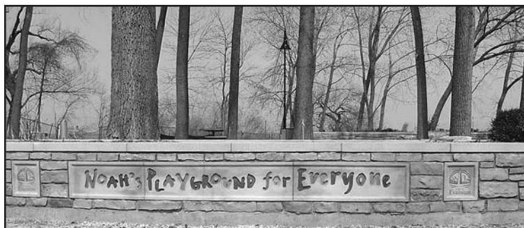
Construction on Noah's Playground for Everyone continued this spring. In mid-April, above, some of the hardscaping was completed. A dedication ceremony is being planned for July 20 at 3:00 p.m.
